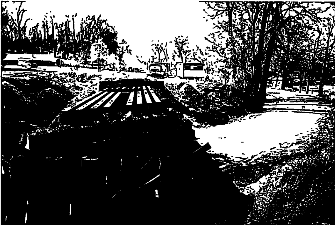
Glass Road Bridge – North Approach – Looking South Showing Trailer, Car Port and Boat Encroaching on Right-of-Way
