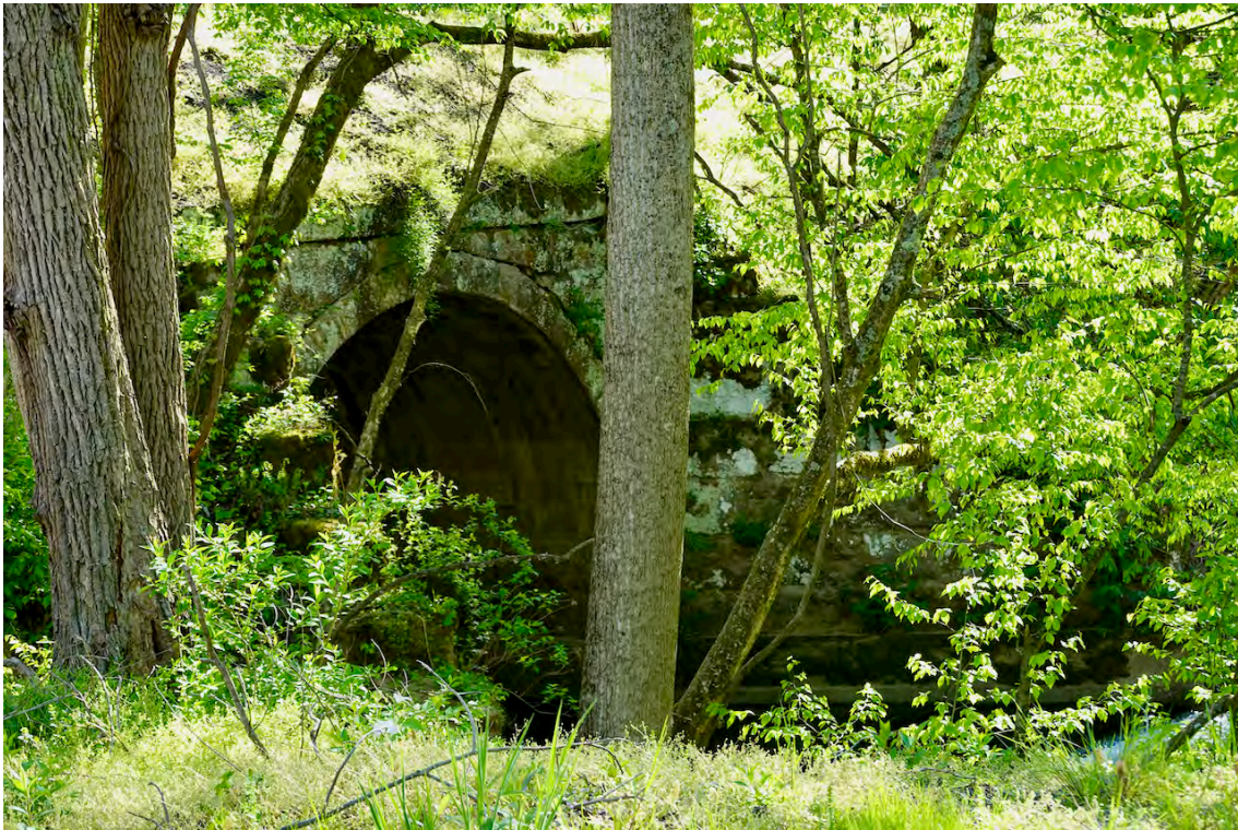
Bridge No. 47/2 Middle Creek (MP 66.85)
