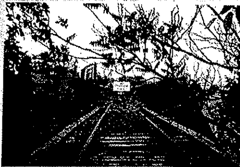
Bridge 2 - Milepost TW 0.62
