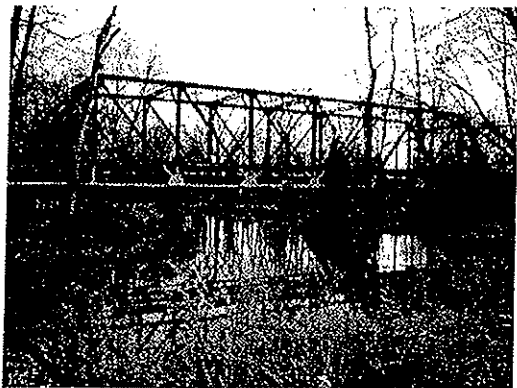
Looking east at the existing bridge
