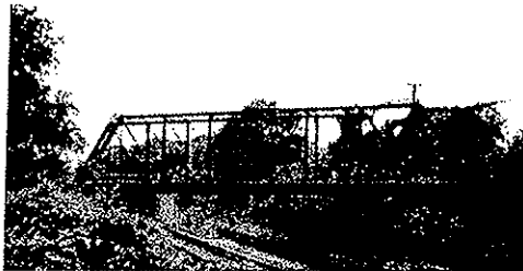
Bridge 3 - Milepost TW 0.99
