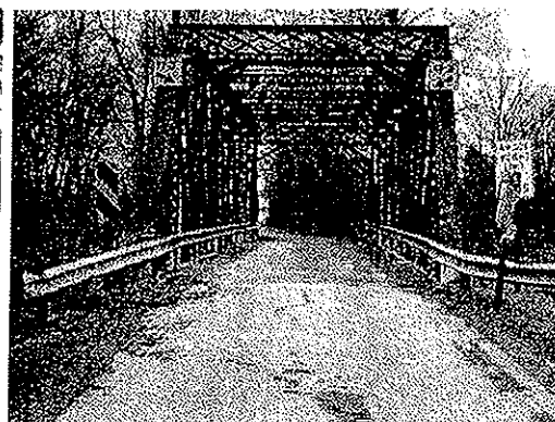
Looking north at the existing bridge
