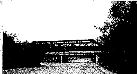
Bridge 2 - Milepost TW 0.62
