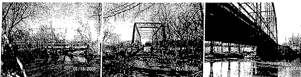
3 Views of the Caldwell Road Bridge in Crawford County
