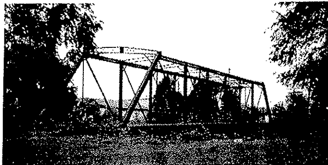
Bridge 3 - Milepost TW 0.99
