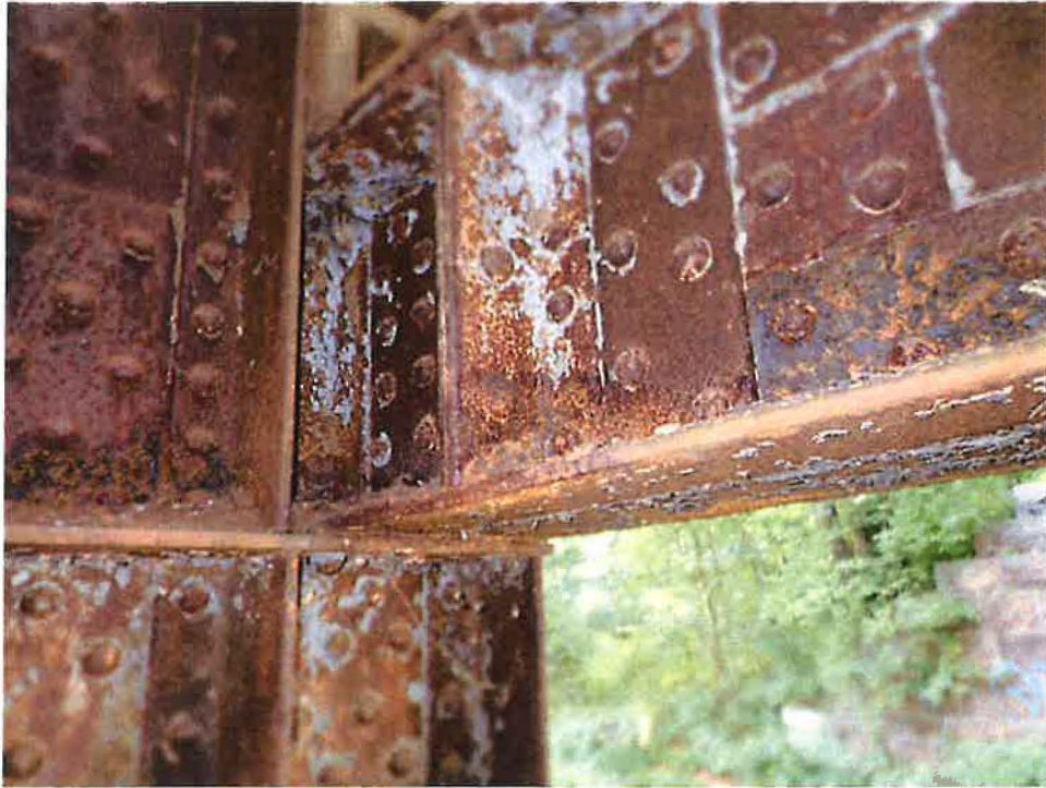
Photo 11: Rusting of riveted steel panels above the bridge pier
