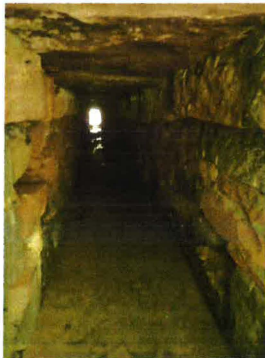
Photo 24: Interior of Culvert 3
