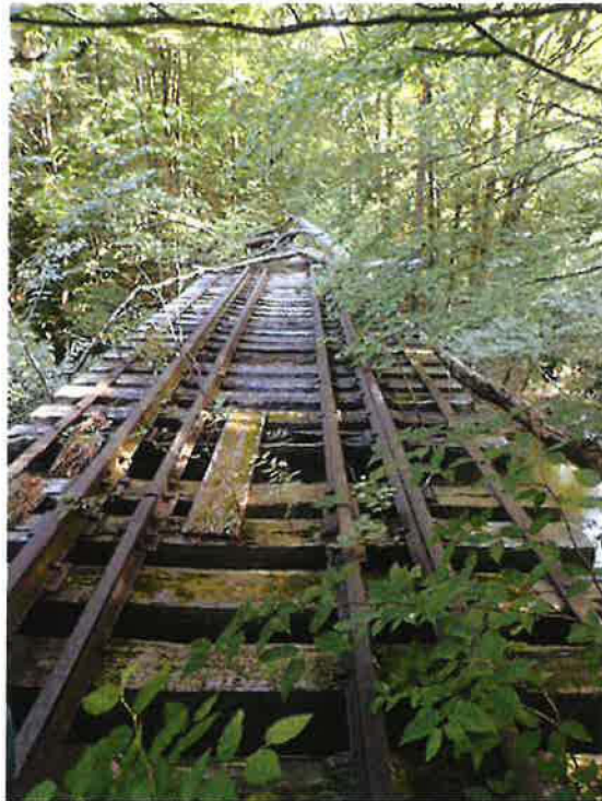
Photo 7: Existing timber deck with railroad ties
