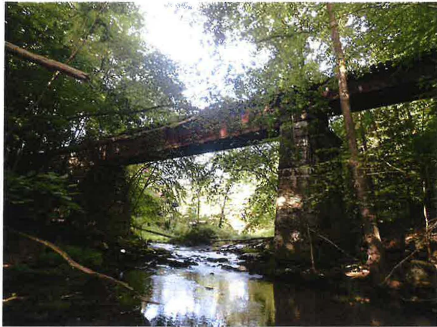
Photo 1: East Elevation of the Manhan River Bridge
