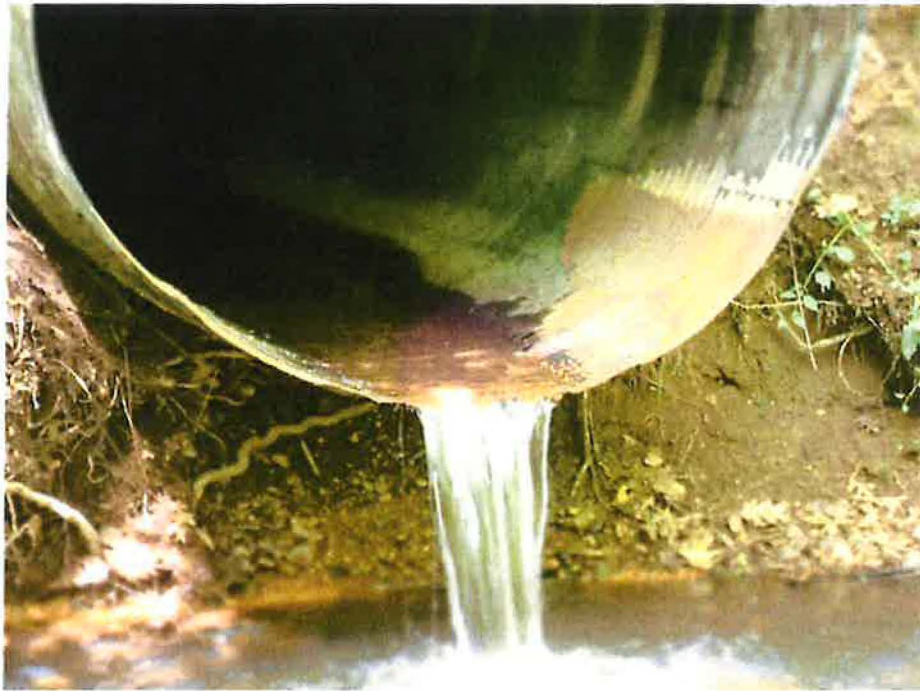
Photo 27: Interior of Culvert 4
