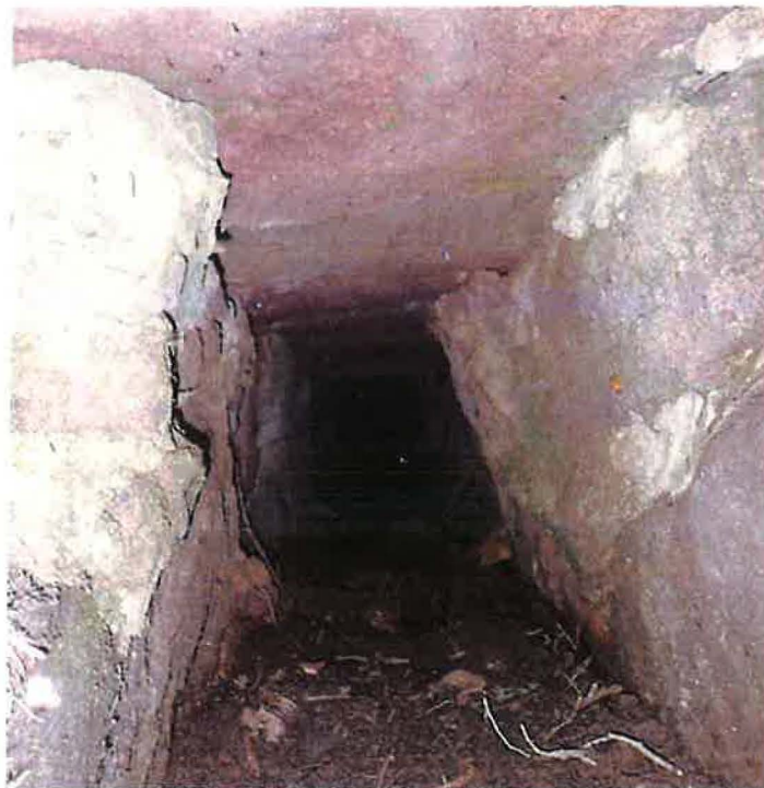
Photo 18: Interior of Culvert 1
