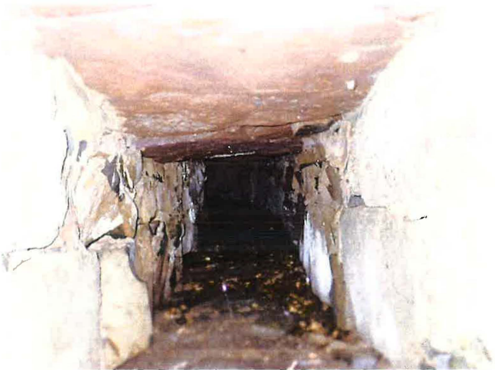
Photo 30: Interior of Culvert 5
