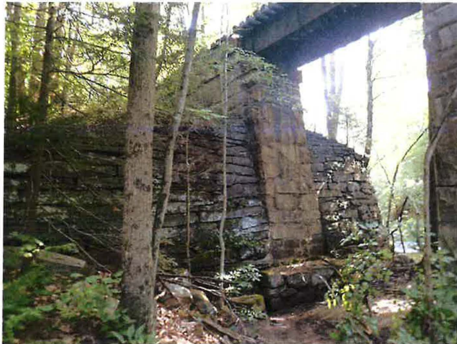
Photo 4: View of the North Abutment
