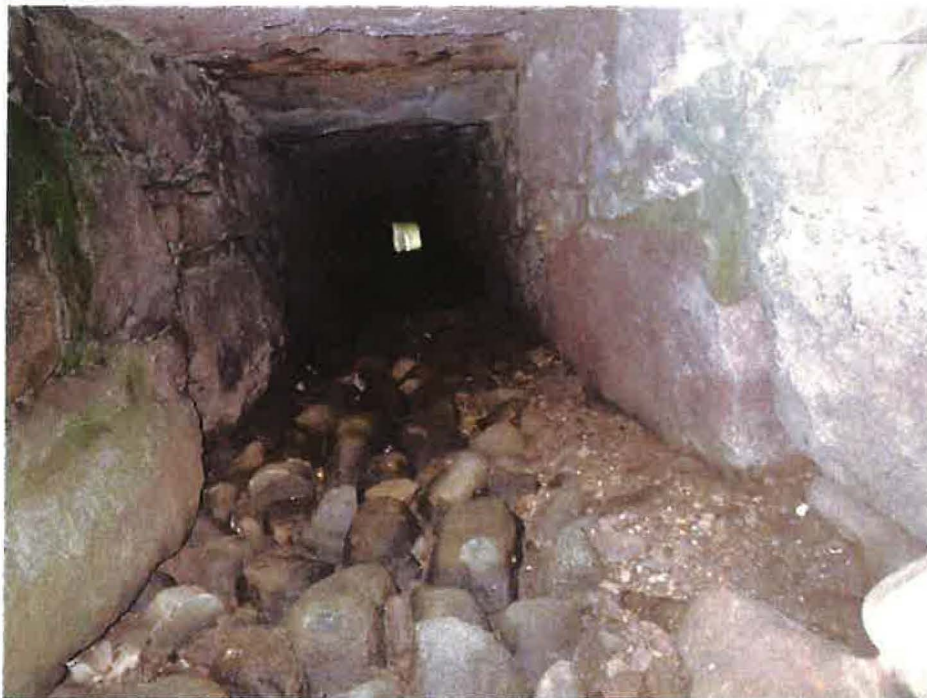
Photo 45: Interior of Culvert 9
