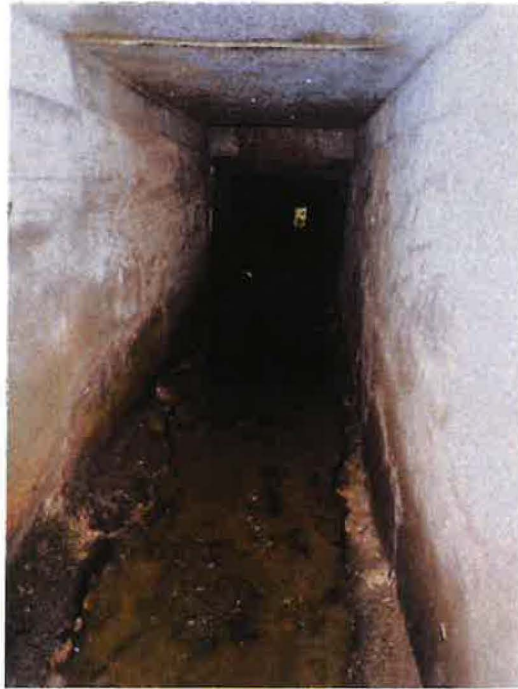
Photo 21: Interior of Culvert 2
