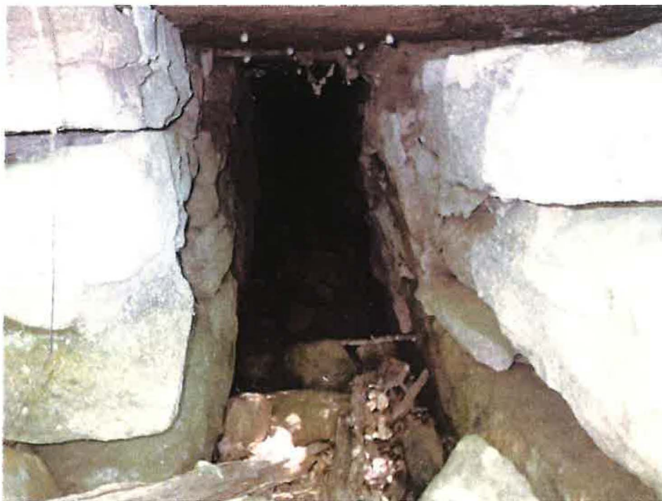
Photo 37: Interior of Culvert 7
