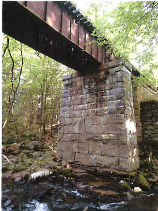
Photo 3: View of the Center Pier
