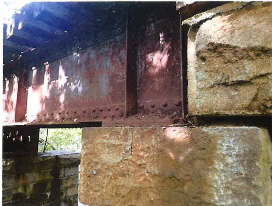
Photo 5: North end of girders, complete section loss of rivet heads
