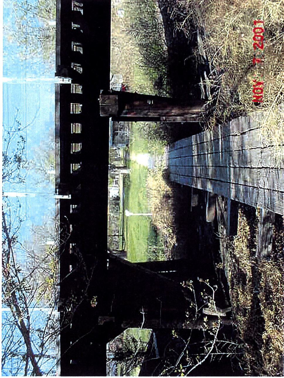
Milepost 42.16 - Built 1930 - Length 42 ft - Height 10 ft - Walkway under Bridge - Open Deck - East Side View.
