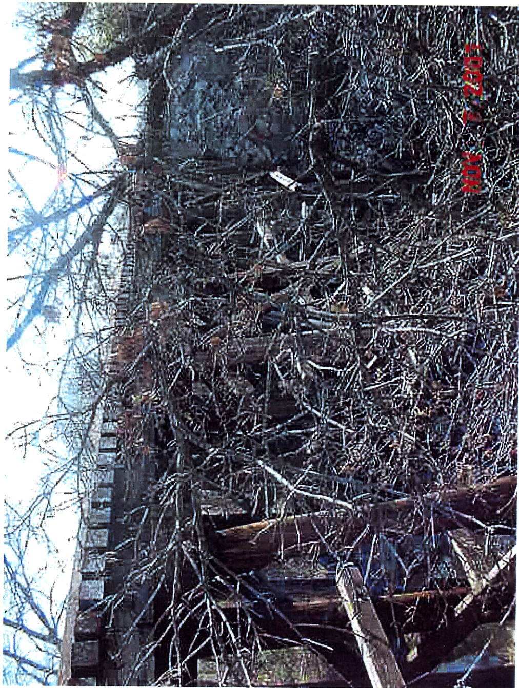
Milepost 41.36 - Built 1931 - Length 119 ft - Height 32 ft - Waterway - Open Deck - 85 lb bolted rail - West side View
