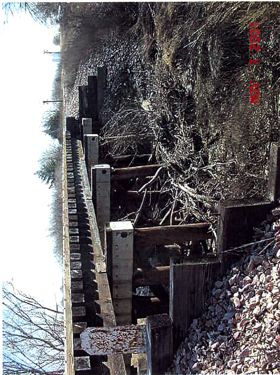
Milepost 39.93 - Built 1923 - Length 56 ft - Height 14 ft - Waterway - Open Deck - 85 lb bolted rail - West Side View
