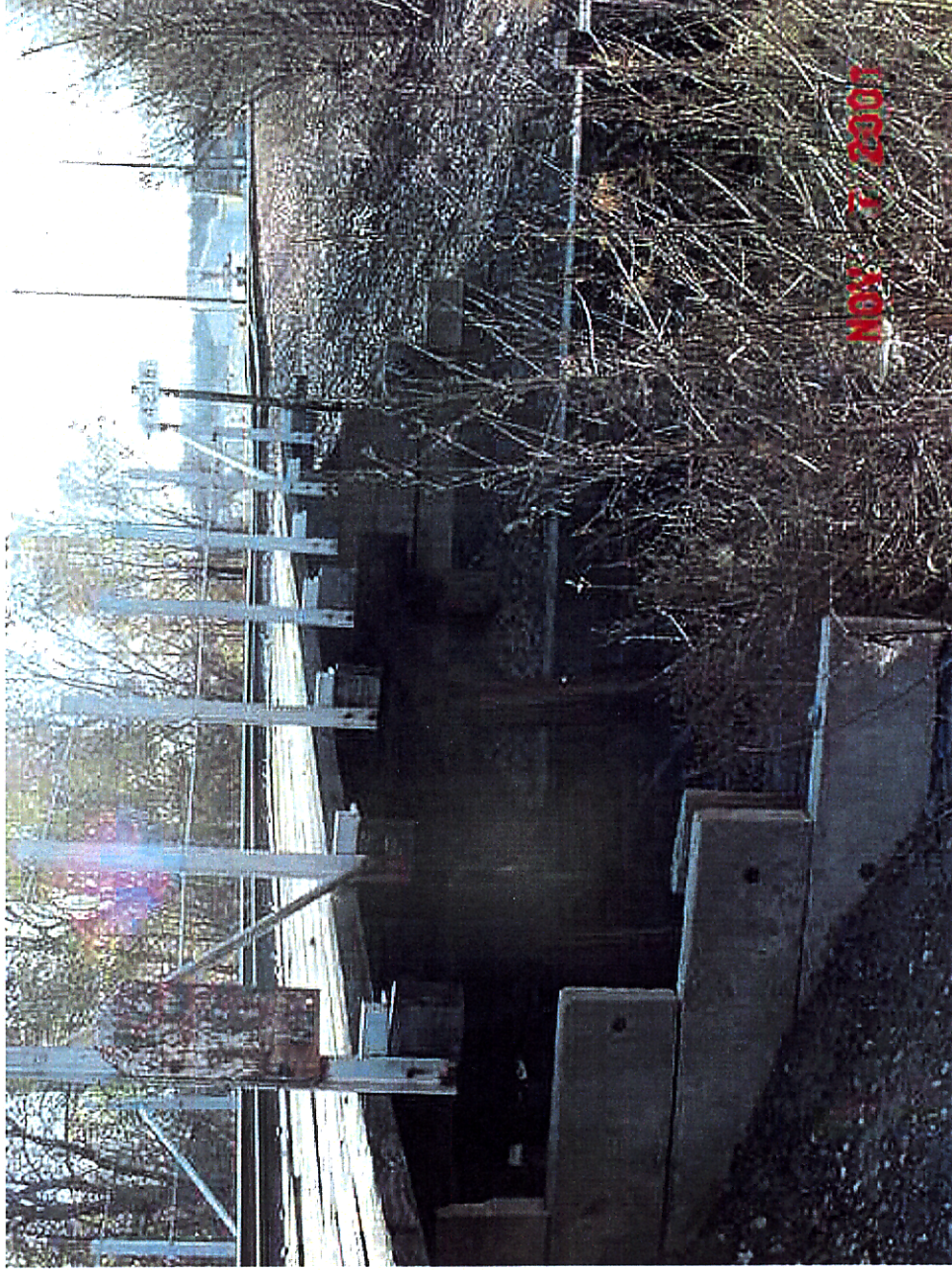
Milepost 42.16 - Built 1930 - Length 42 ft - Height 10 ft - Walkway under Bridge - Open Deck - CWR 112 lb. TR rail - West side View.
