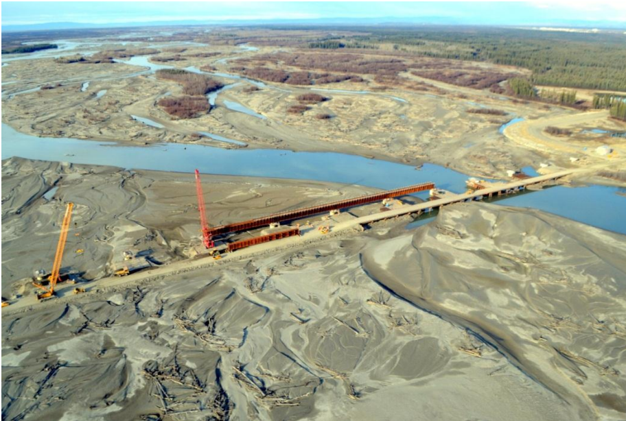
Figure 6. Girder placement. Photographed October 19, 2013.
