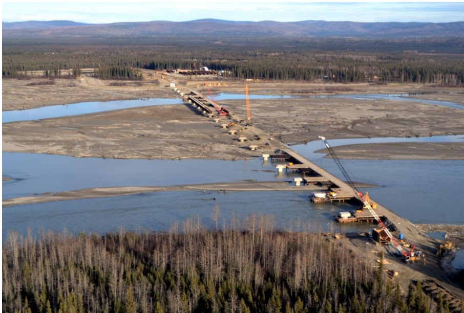
Figure 2. Temporary access and piers . Photographed October 19, 2013.
