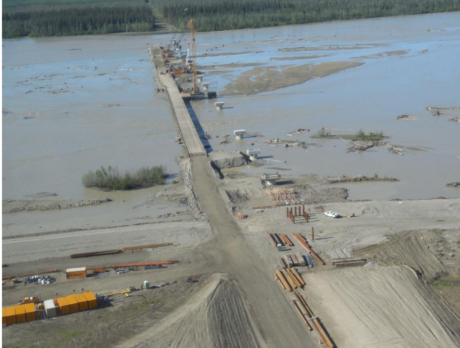
Figure 1. Temporary Access. Photographed July 22, 2013
