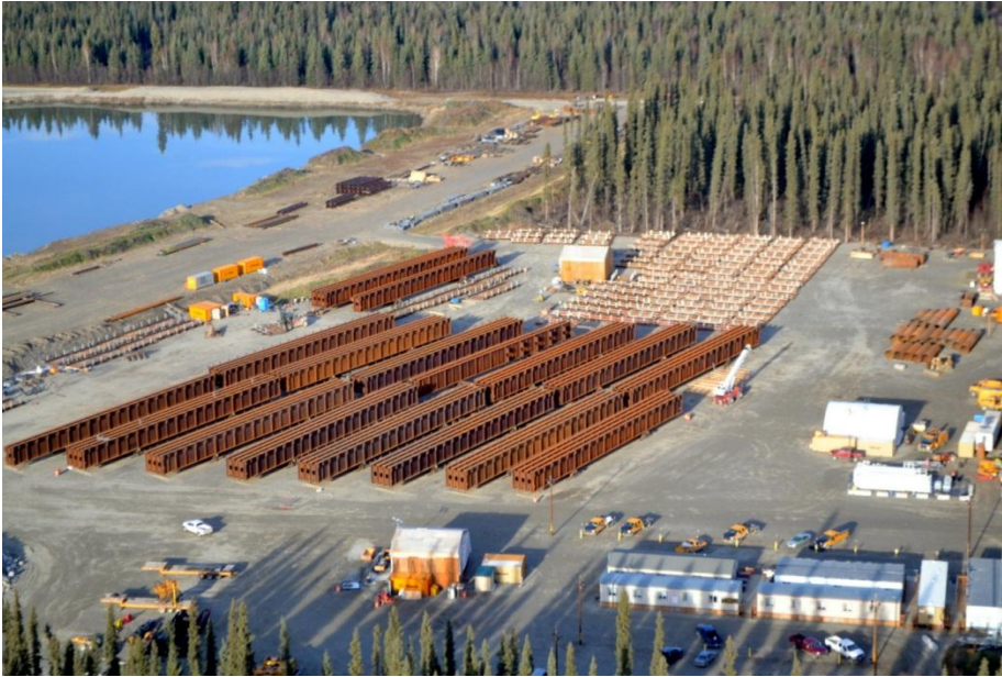
Figure 5. Girder yard. Photographed October 19, 2013
