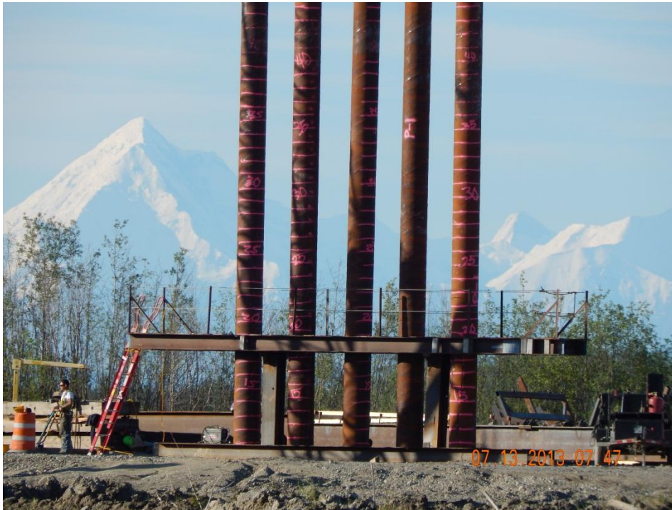
Figure 3. Piles at Abutment 1. Photographed July 13, 2013.
