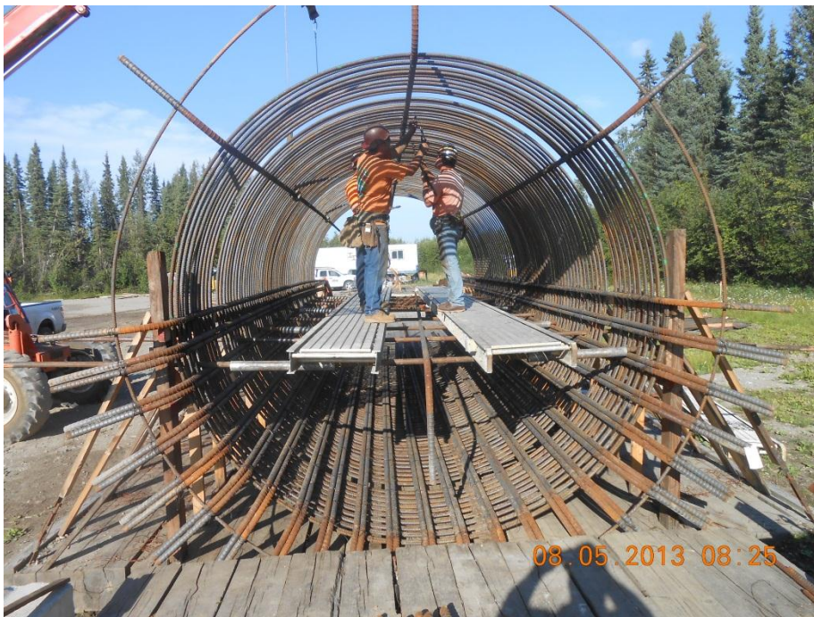
Figure 4. Construction of 12' rebar cage. Photographed August 5, 2013
