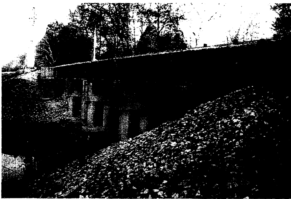
BRIDGE NO. 163.5 - EAST SIDE
