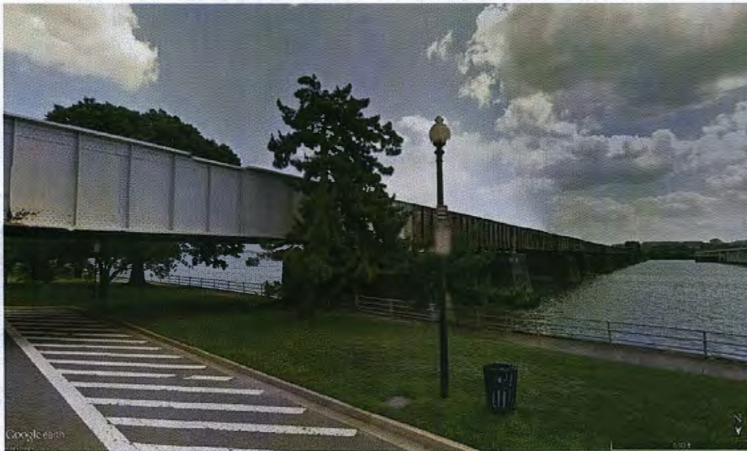
This is a view of the rail bridge over the Potomac River, taken from Ohio Drive in Washington DC.
