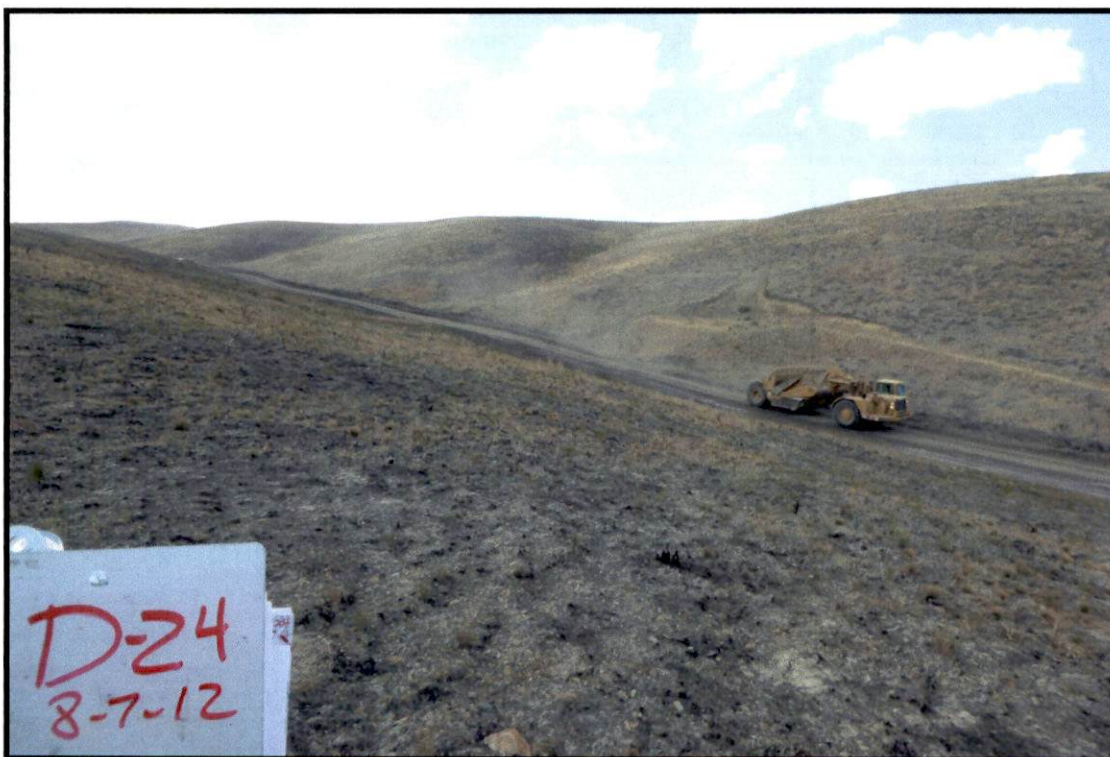
Photo A24: Looking upgradient at DP-24 along Drainage 24. Drainage is now used as a haul road.
