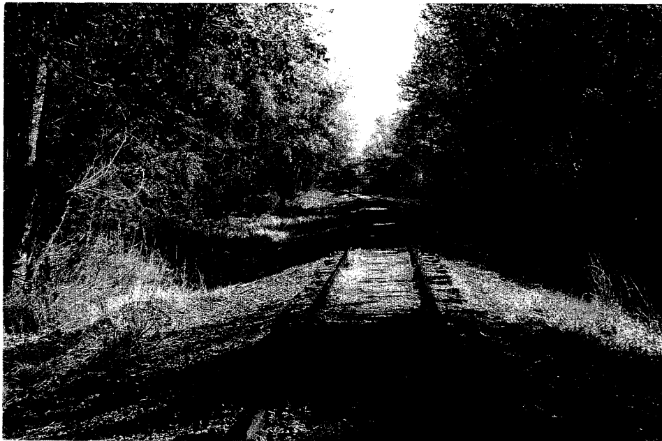
No. 18: Looking north 1000' north of Country Club Road
