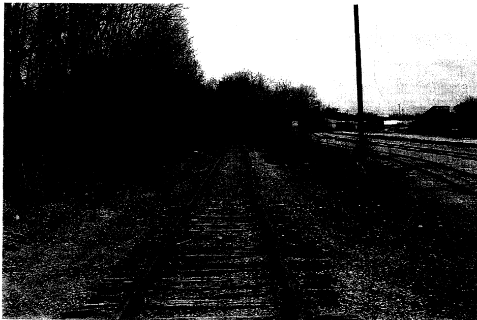
No. 8: At the connecting track switch with CSXT looking north
