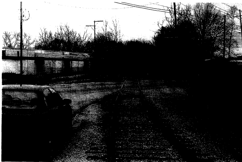
No. 2: At Rogers Street looking S.E. along the "Warehouse Track"
