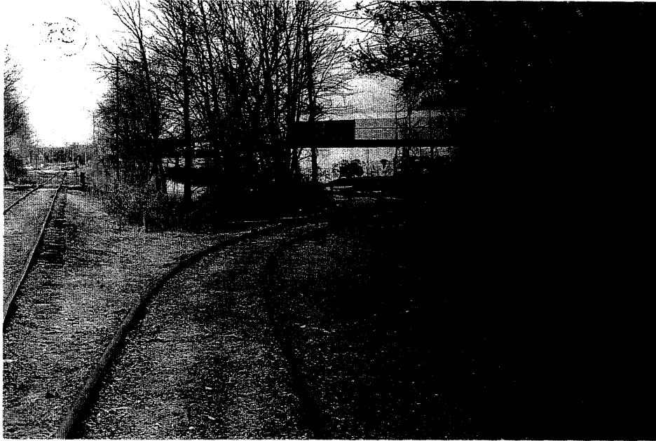
No. 3: At the switch to Indiana Warehouse looking north. Main is on the left.
