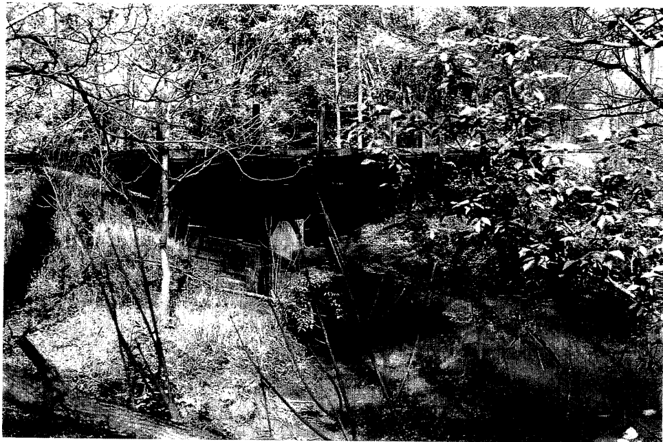
No. 22: Bridge at XA-1.8 (Shown on Map attached as Exhibit B-1)
