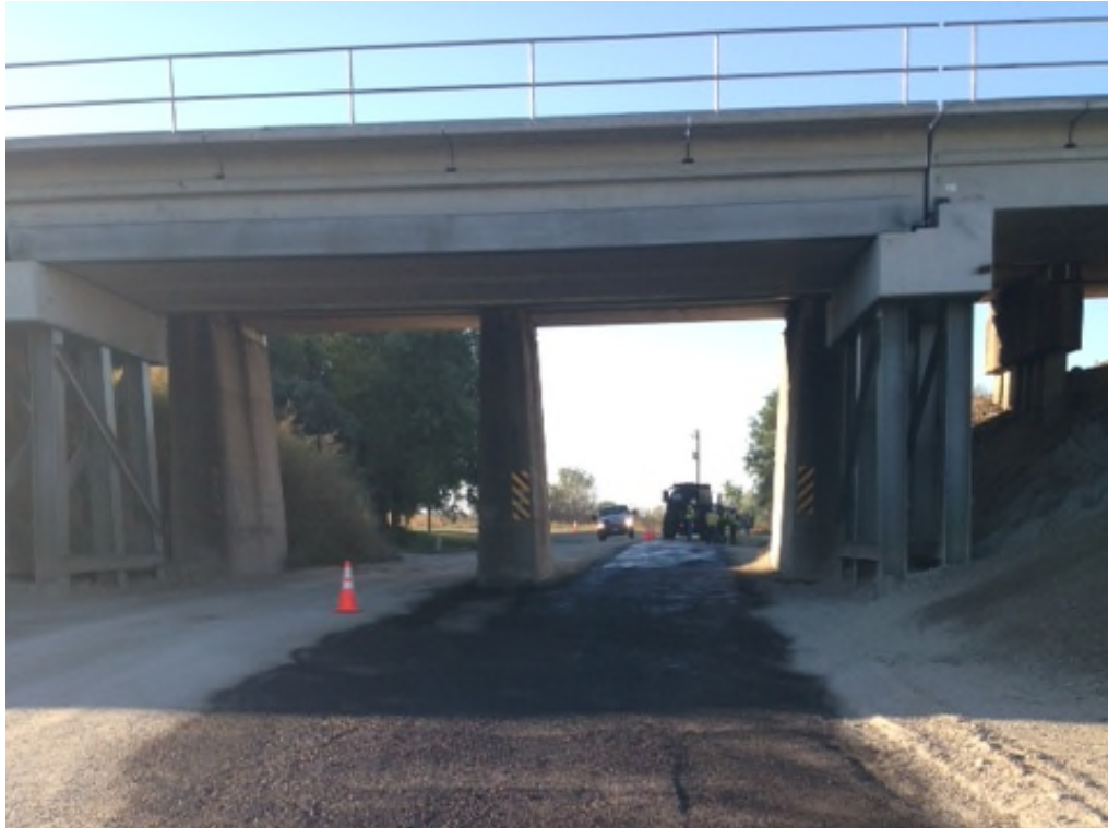
Figure 3 – Precast Concrete Box Span Bridge Photo
