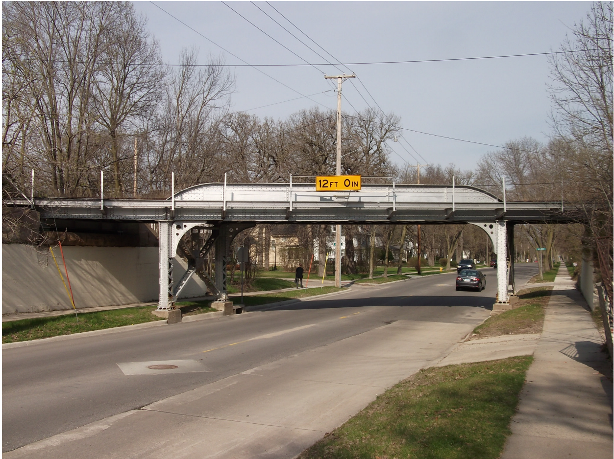
Structure 2: State Street, MP 156.15, constructed 1902.
