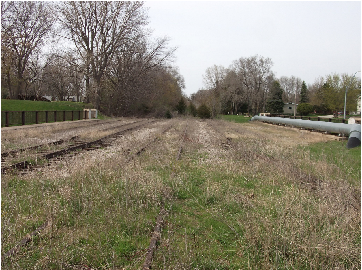
Structure 3: Hwy 122 / 5th St - MP 156.45, constructed 1958
