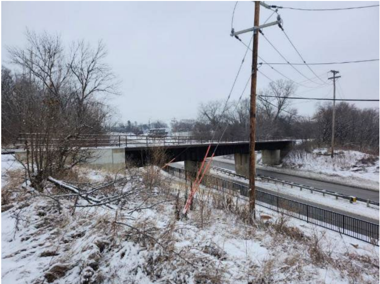
Facing East at side of the bridge
