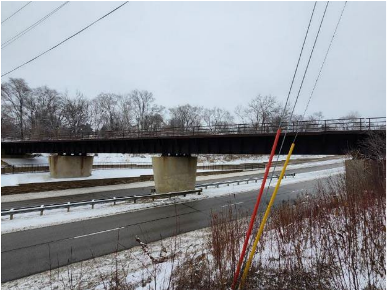
Facing Northeast at side of the bridge
