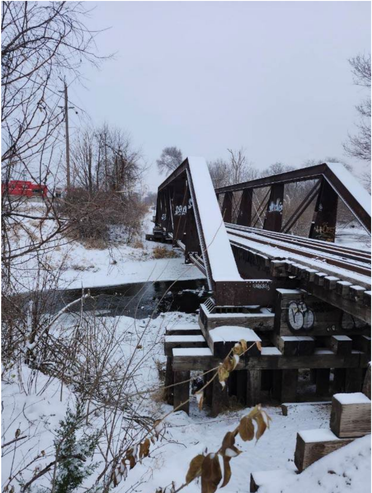
Facing Northwest along the side of the bridge
