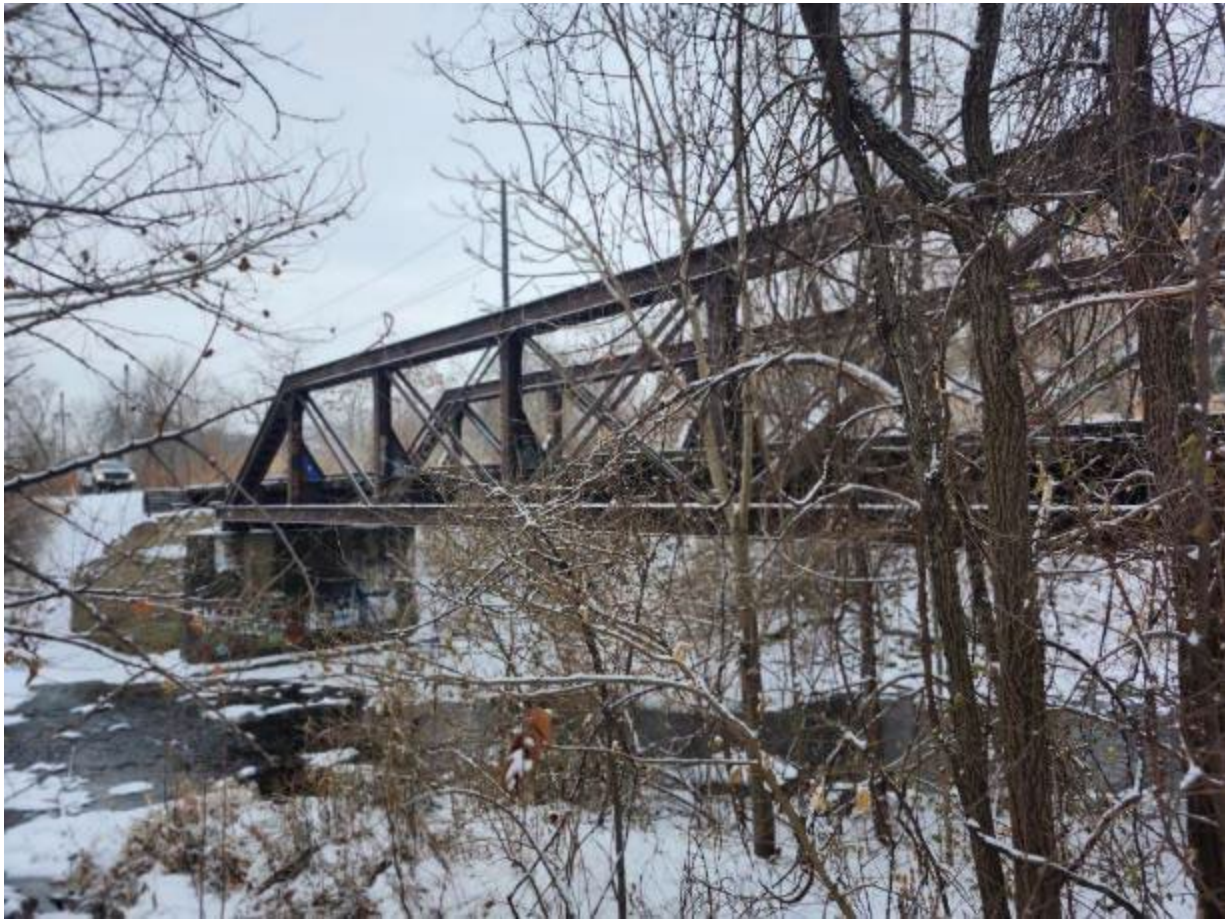
Facing North at side of the bridge
