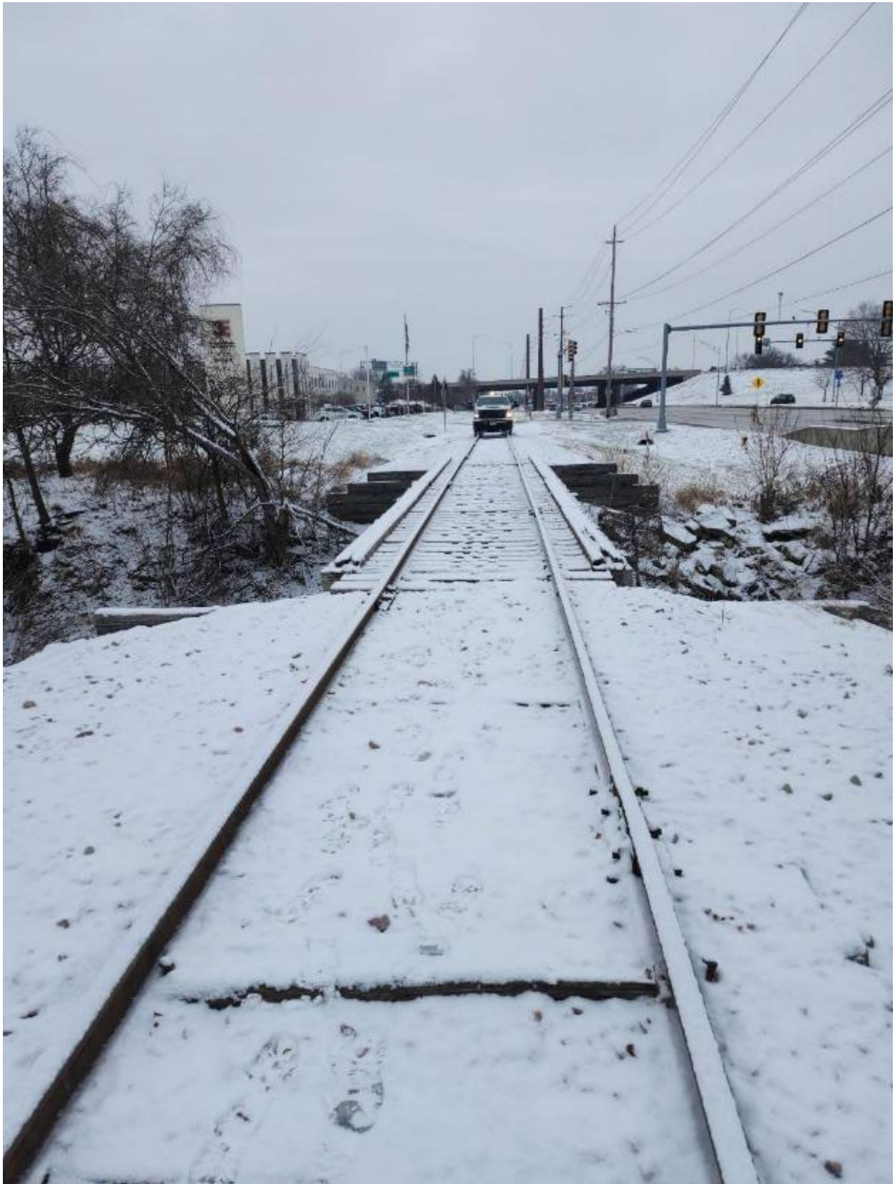
Facing Southeast along the tracks
