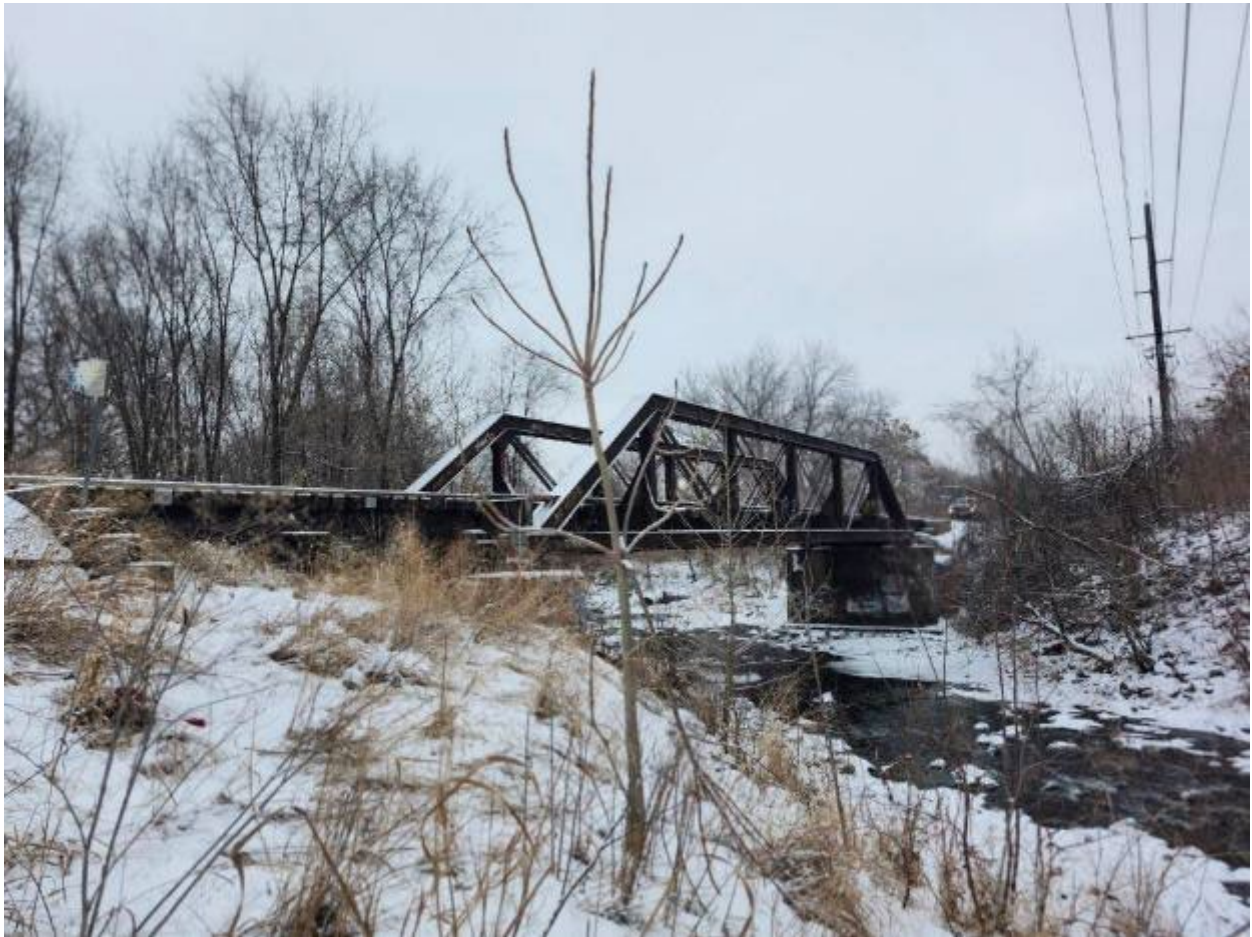
Facing East at side of the bridge
