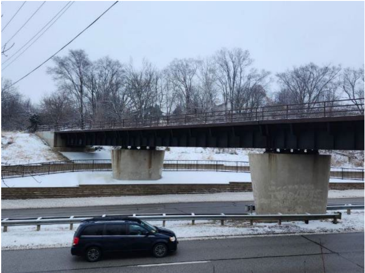
Facing North at side of the bridge
