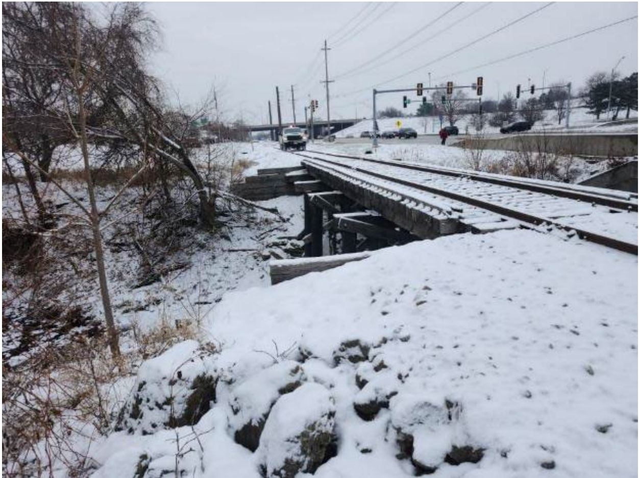
Facing South at side of the bridge
