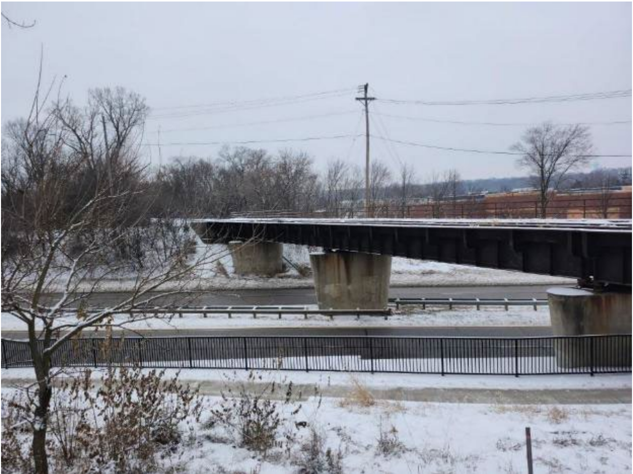
Facing South at side of the bridge
