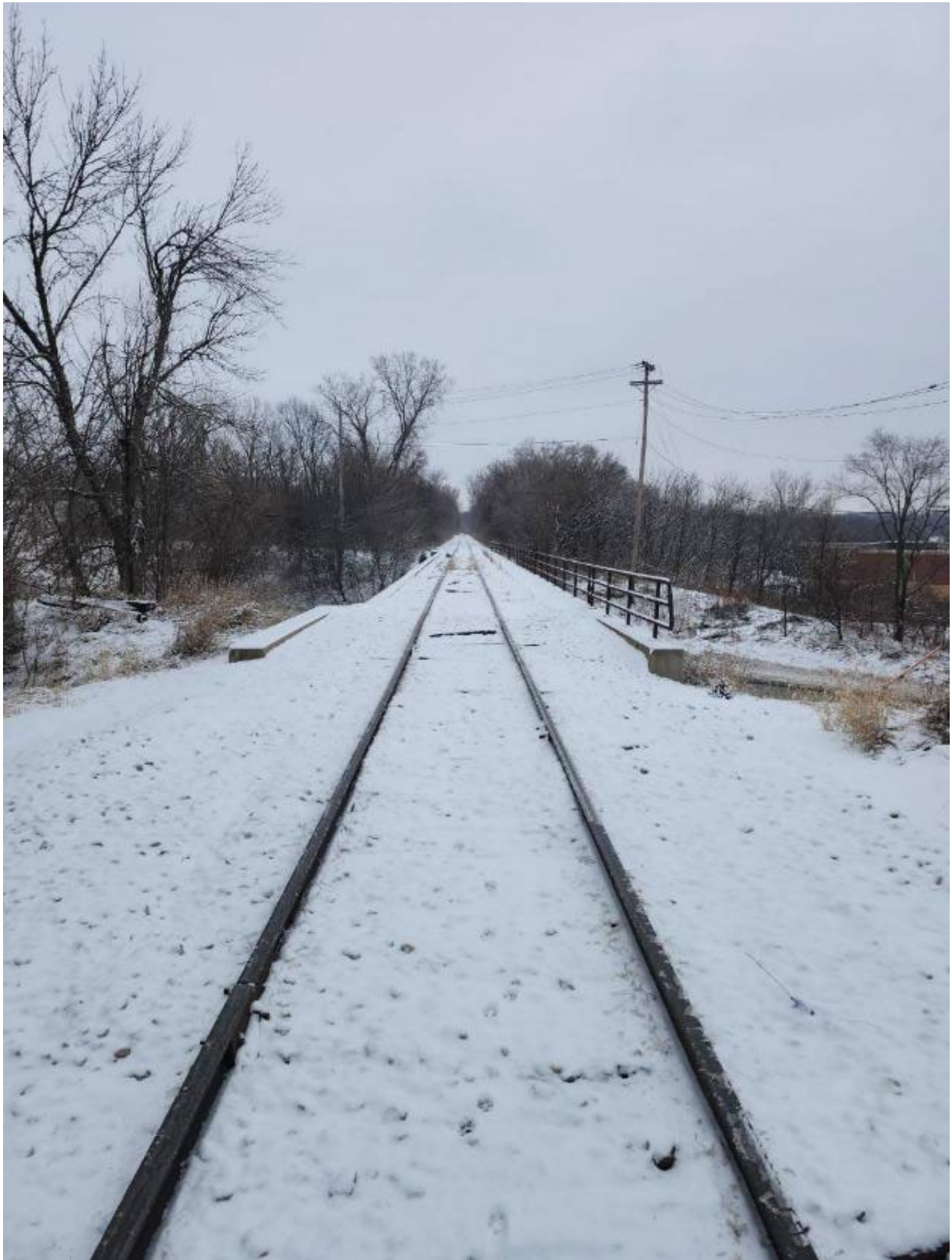
Facing Southeast along the tracks
