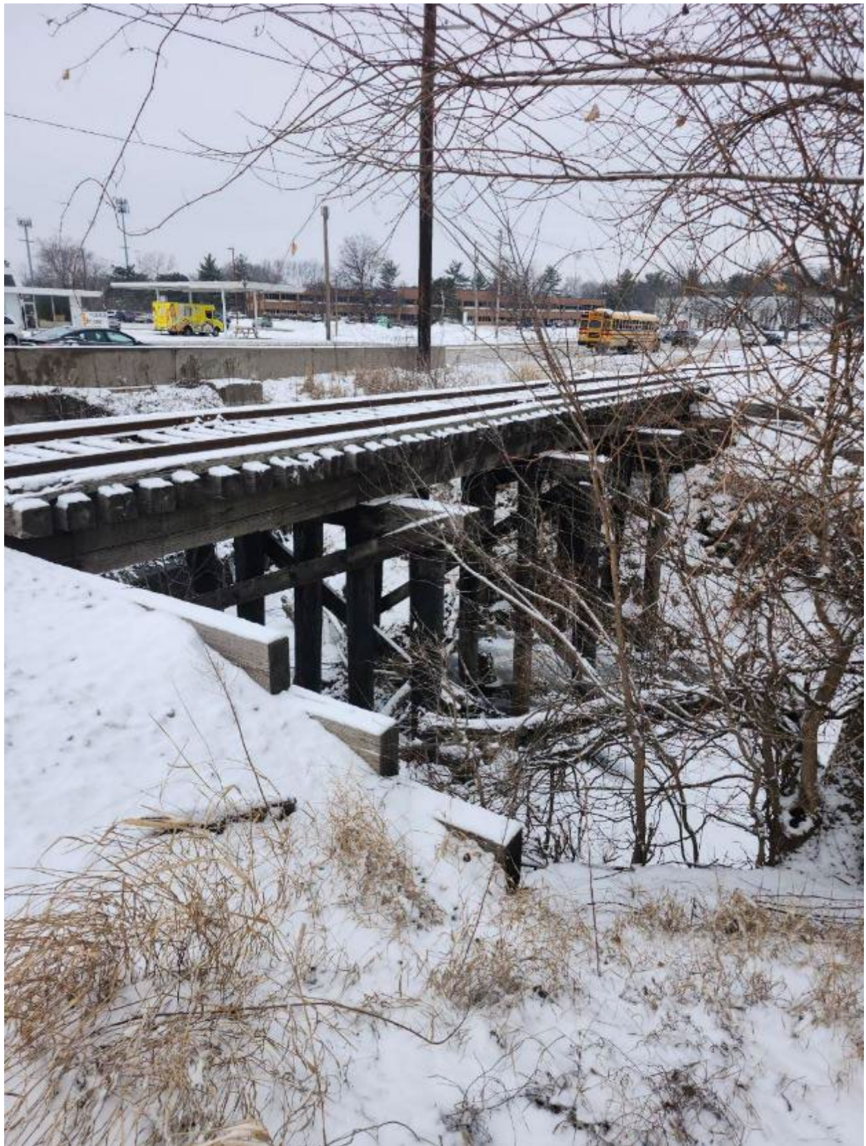
Facing West at side of the bridge
