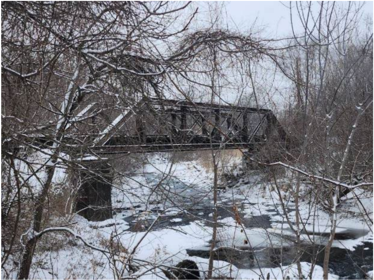
Facing West at side of the bridge
