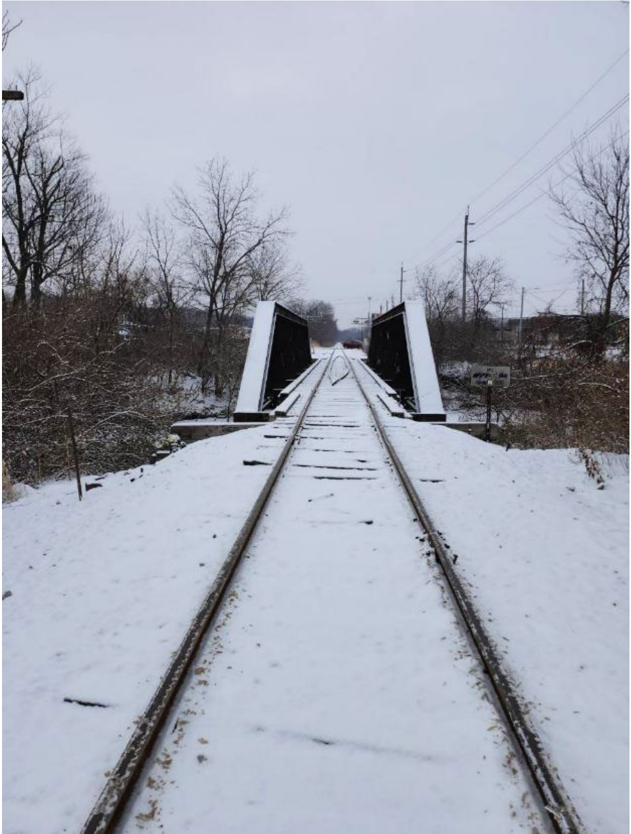
Facing Southeast along the tracks
