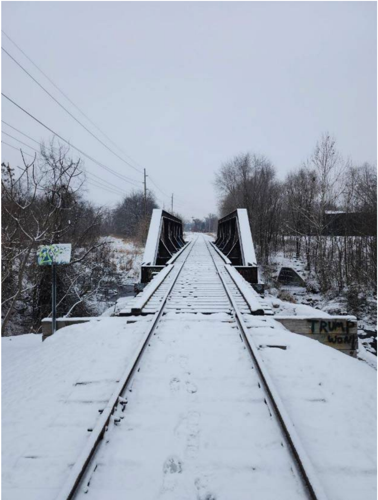
Facing Northwest along the tracks
