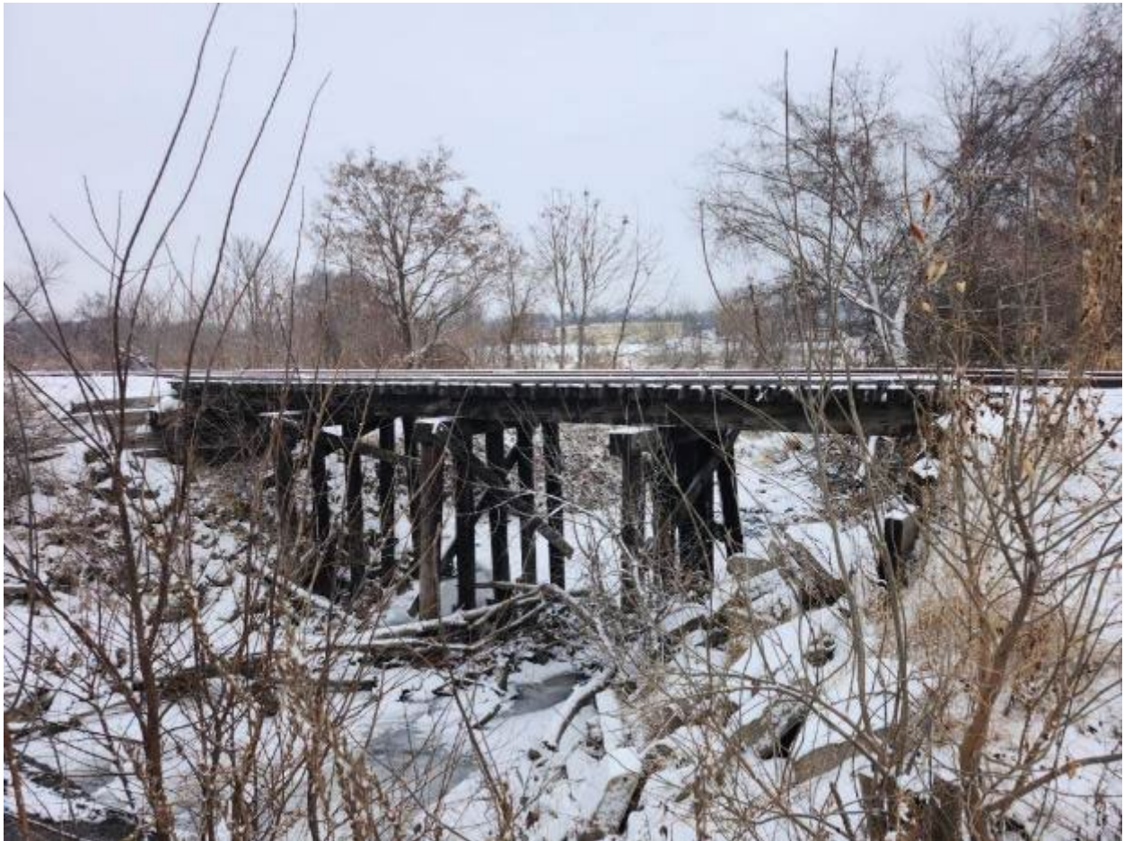
Facing Northeast at side of the bridge
