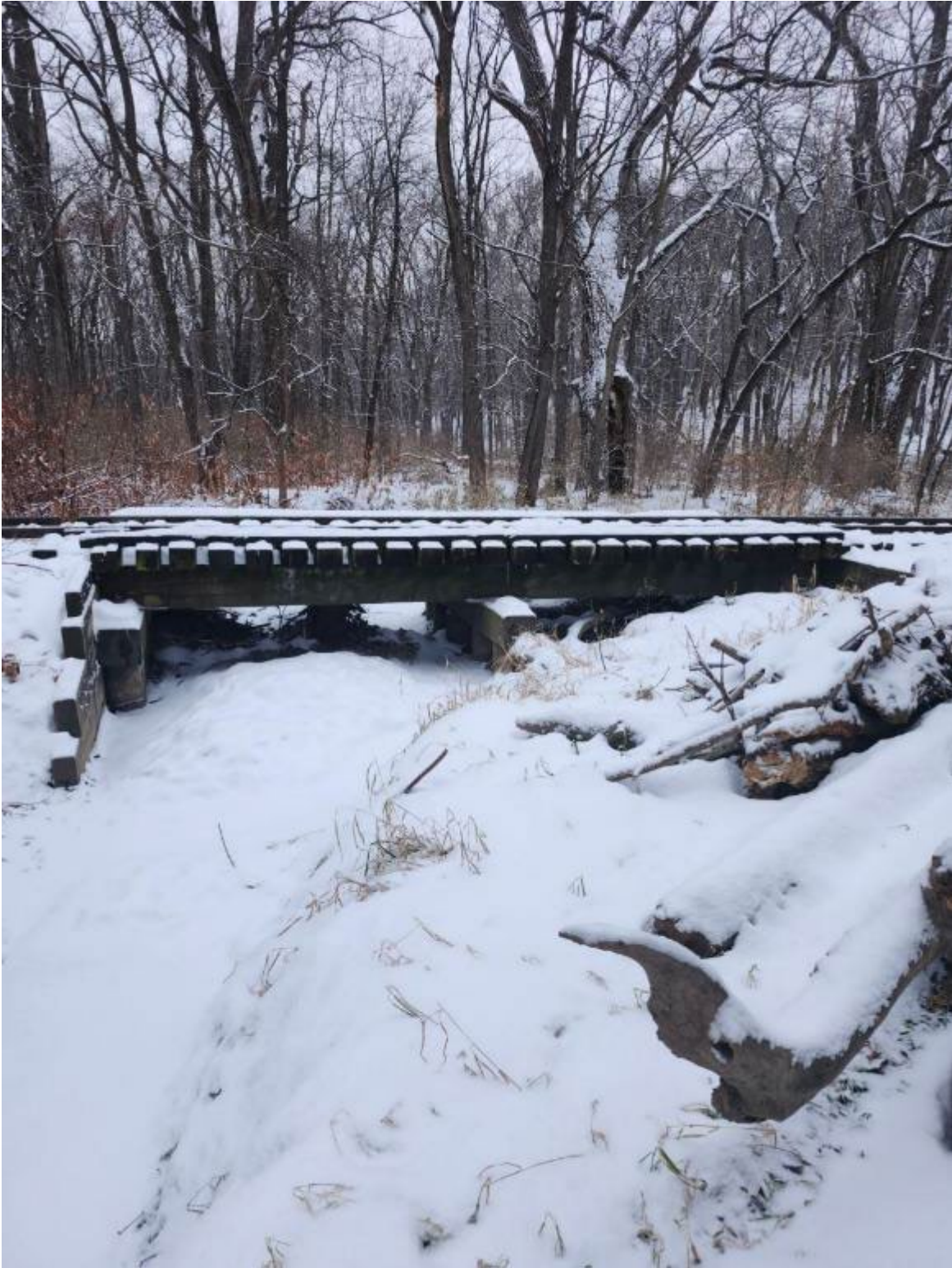
Facing Southwest towards side of the bridge
