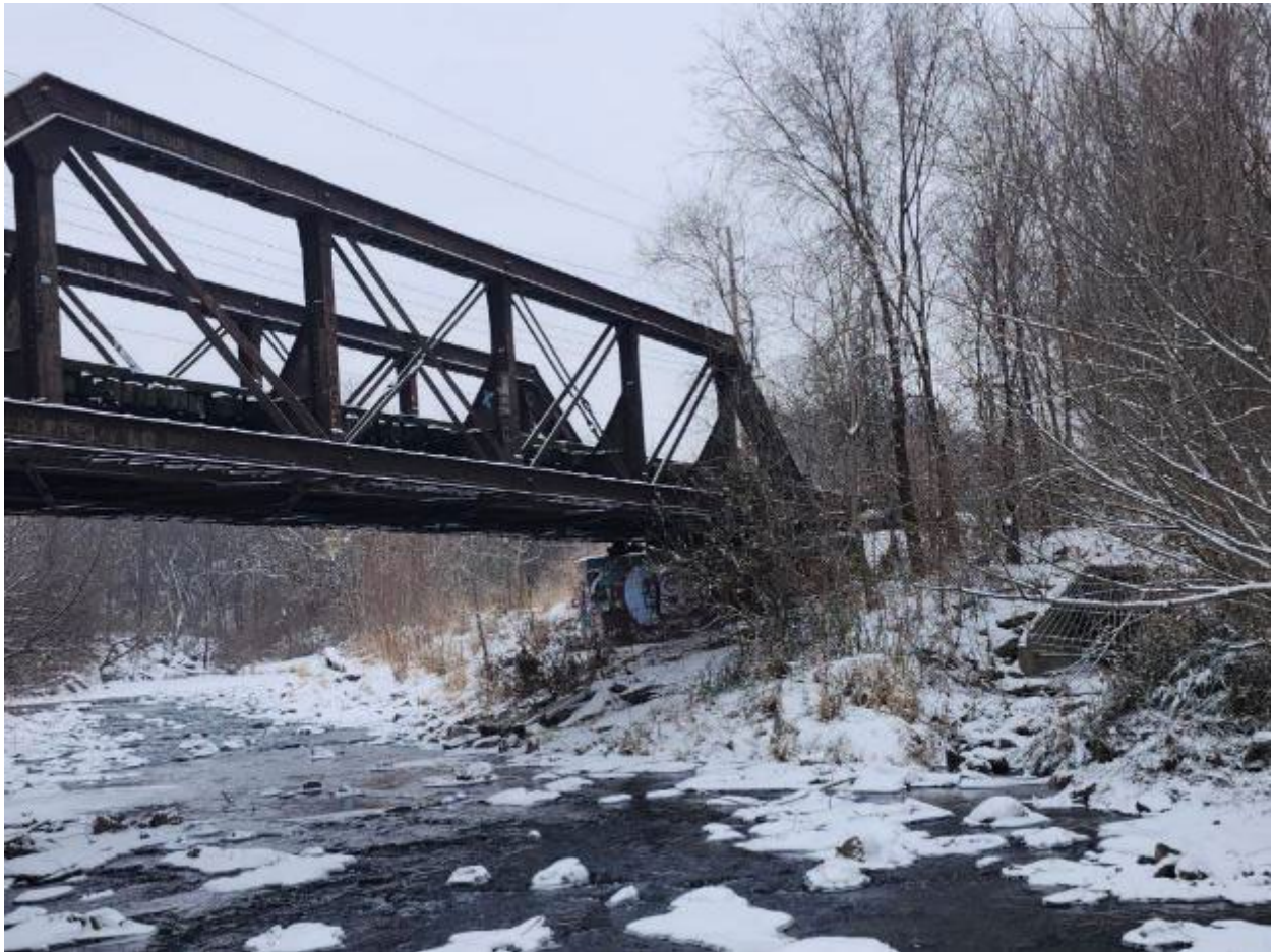
Facing West at side of the bridge
