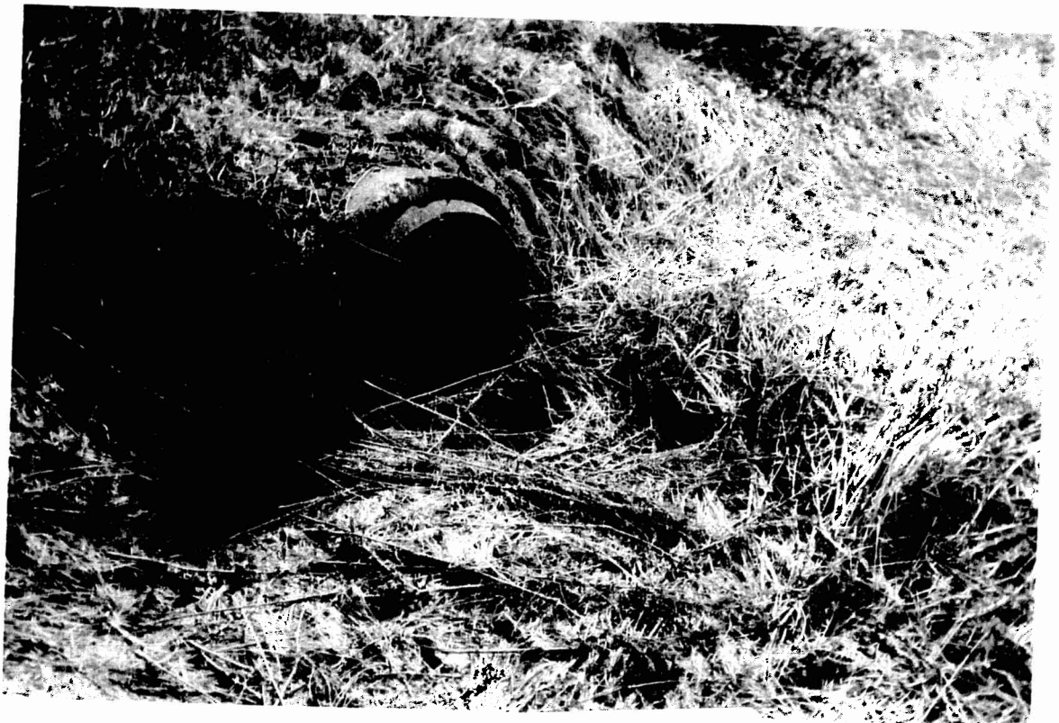
21. MP 387.9 Adventure Creek U778.5 – Concrete Pipe Culv. 24"
