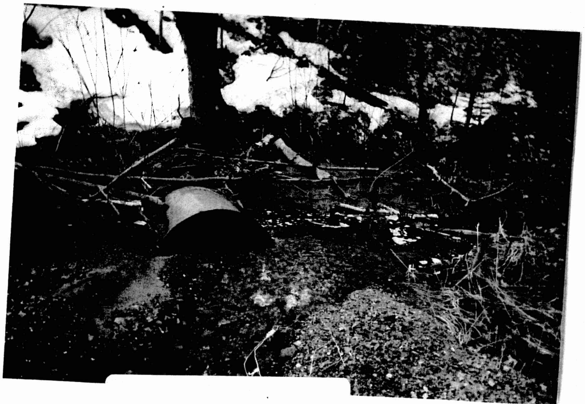
39. MP 396.5 Ontonagon River U833- Iron Pipe Culv. 30"
