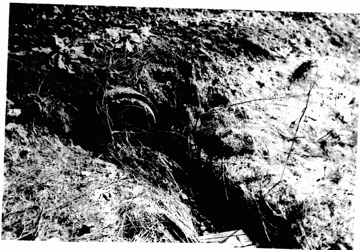
24. MP 388.5 Adventure Creek U781.5 – Concrete Pipe Culv. 30"
