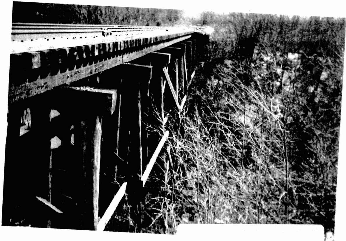
25. MP 388.6 Adventure Creek U672 - Pile Trestle 9 span 126'
