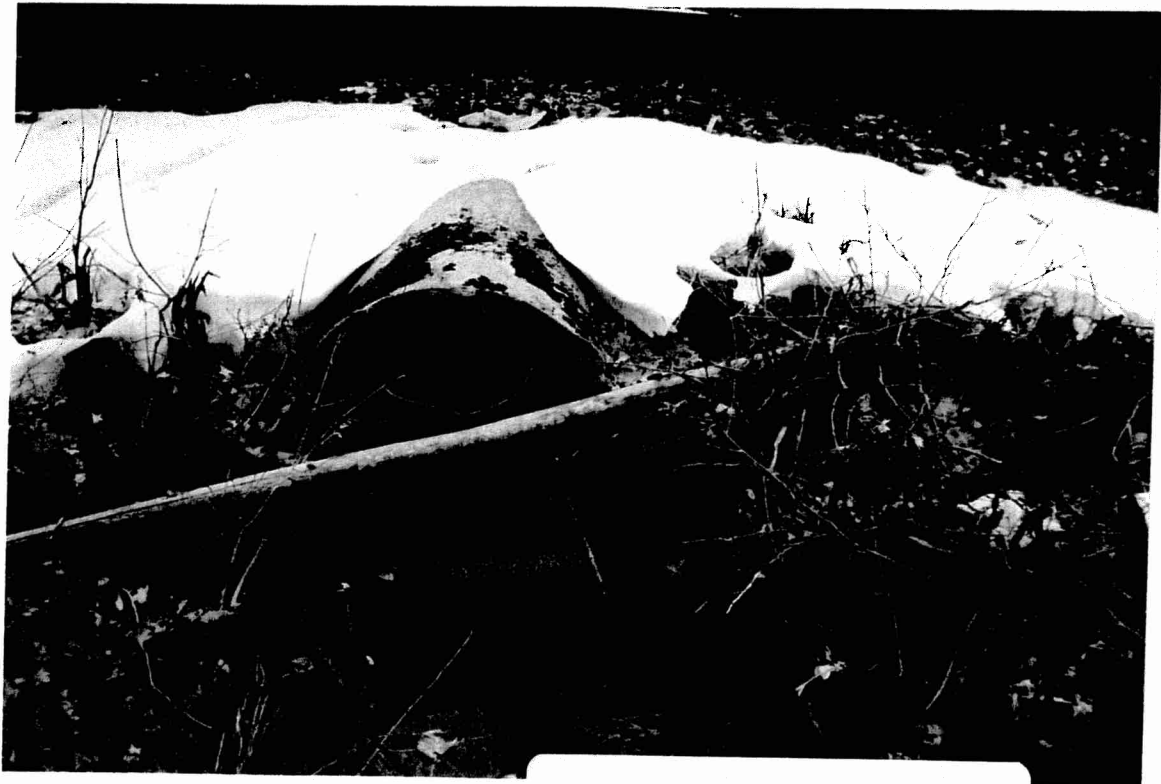
4. MP 374.5 Burritts Creek U652 – Concrete Pipe 36"
