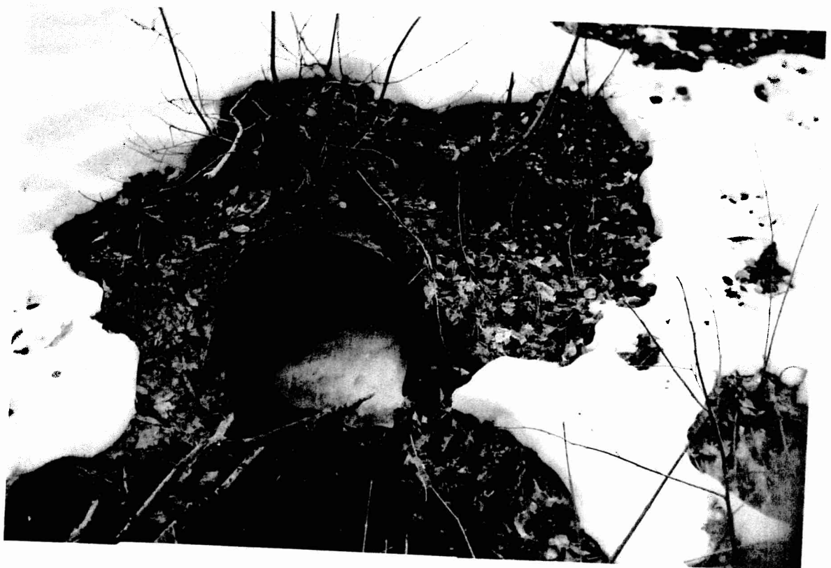
38. MP 396.0 Ontonagon River U682- Iron Pipe Culv. 36"
