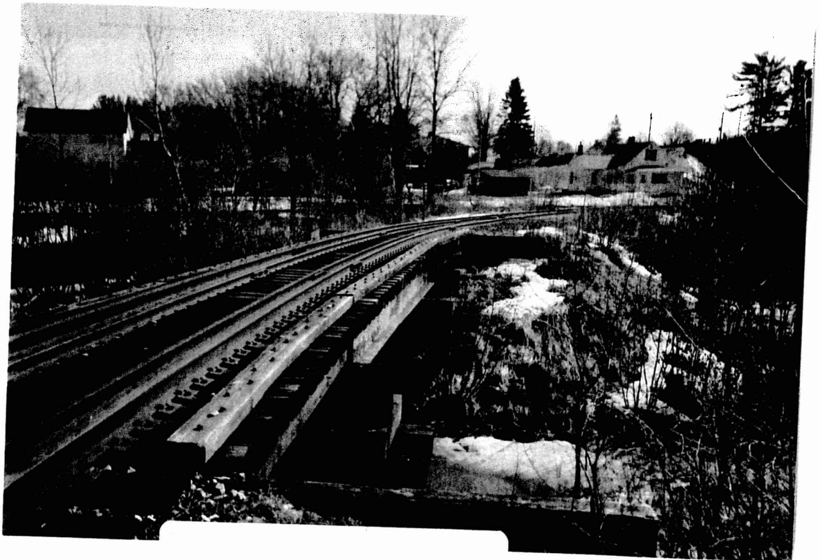
48. MP 407.9 Ontonagon River U1800A - 28' Steel Span
