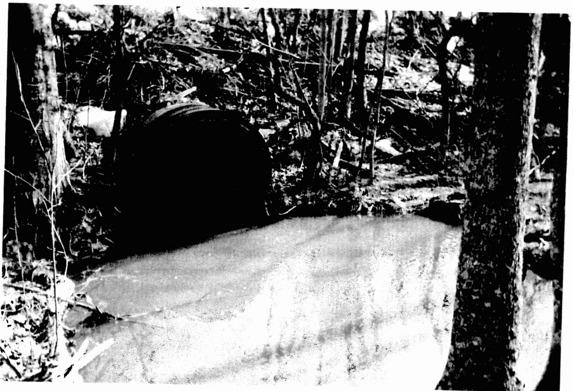
20. MP 387.5 Adventure Creek U778.5 – Concrete Pipe Culv. 24"
