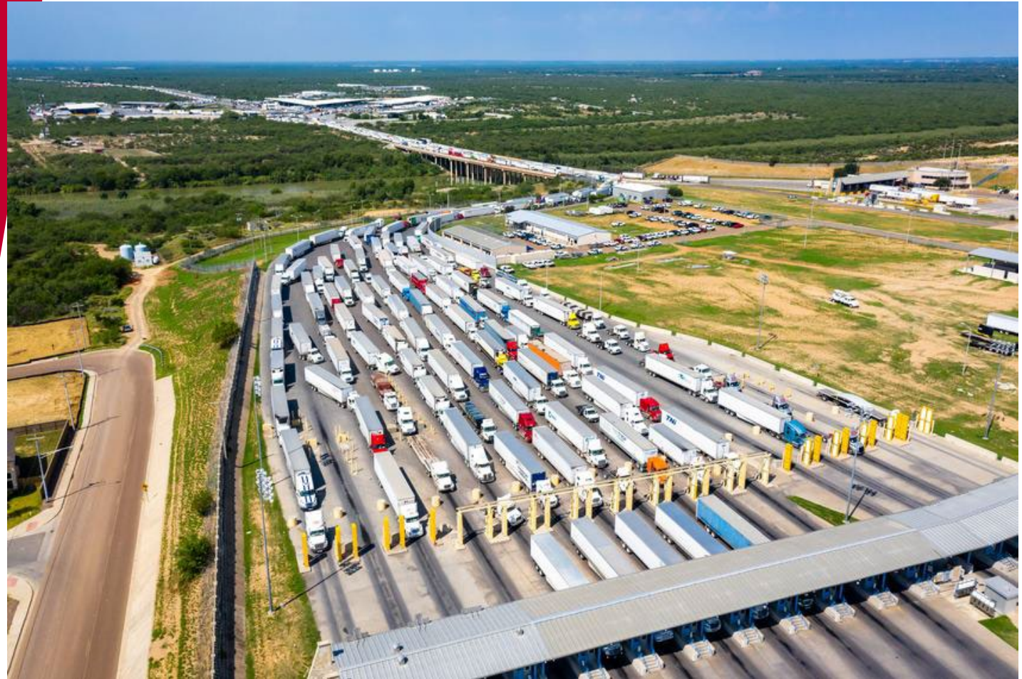
World Trade Bridge at Laredo Gateway ~1.8M trucks annually, or ~5,000+ per day
