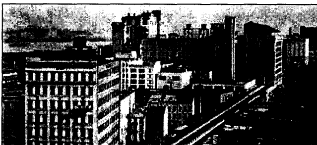
A view of the viaduct looking north from Clarkson Street, with tracks passing through two buildings
