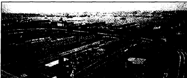
General view of 30th Street Yard, showing it encircled by new viaduct which loops around
