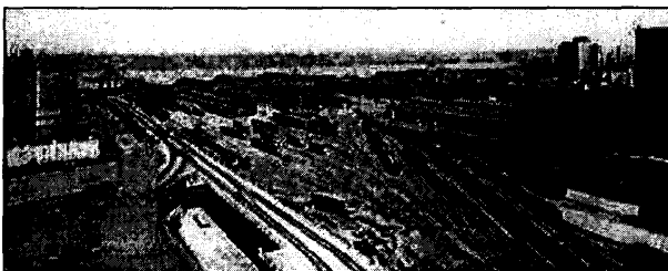
View of the new viaduct at the southwestern side of the 30th Street Yards. This yard is to be reconstructed and improved.
