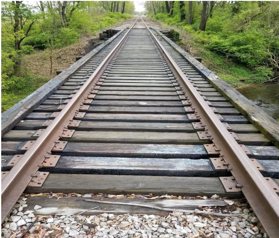
Bridge at milepost 10.6
