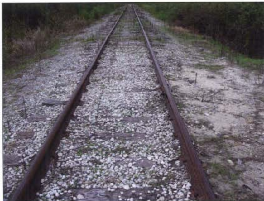
Figure 44. Photograph of railroad tracks in northern portion of project area, facing south.
