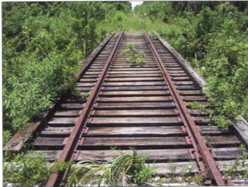
Figure 63. Deck of 8SO5310, facing south.
