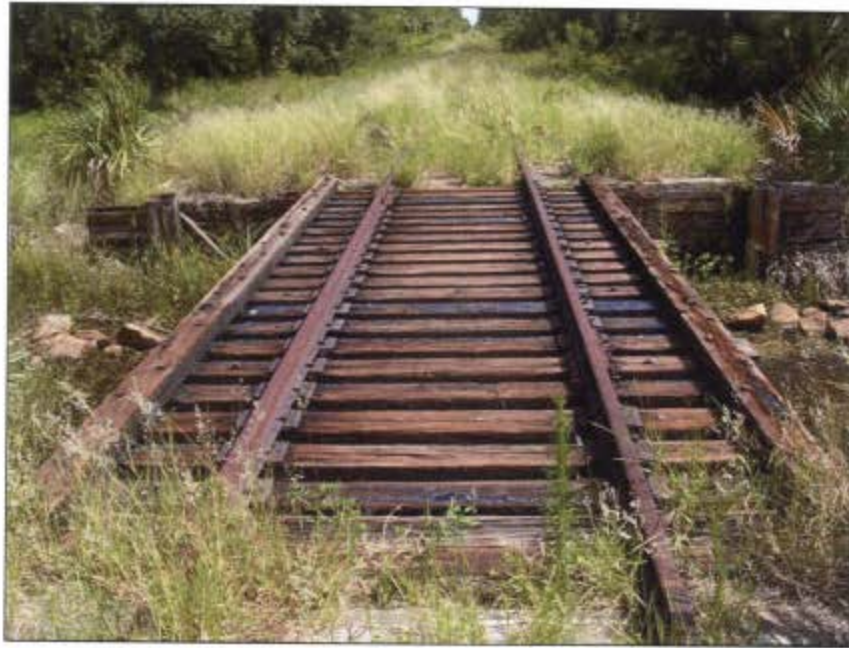
Figure 14. Photograph of the south-central portion of the project area (Bridge 8SO5315), facing north.
