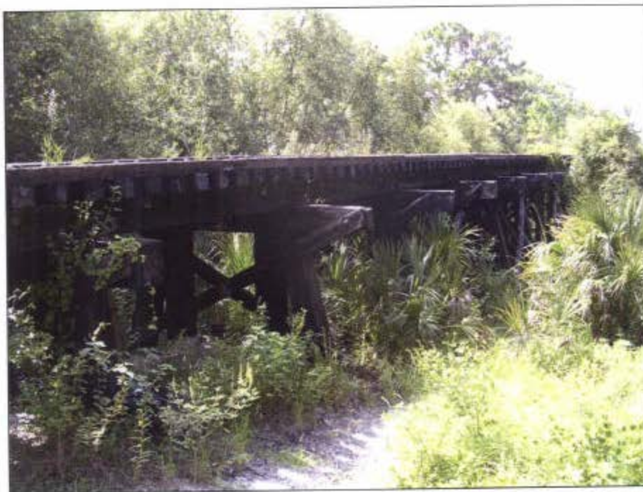
Figure 69. Braced bents with square piles of 8SO5313, with little or no water running underneath the bridge, facing southeast.
