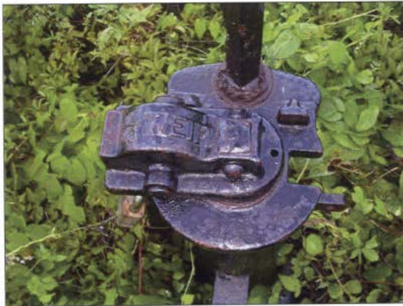
Figure 34. Close up photograph of railroad switch #1.
