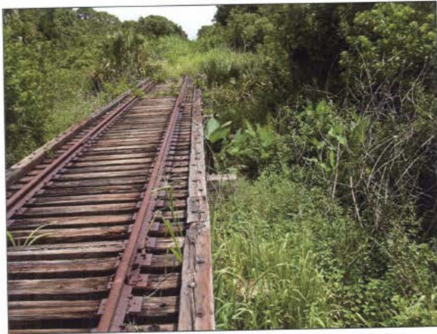
Figure 65. Deck of 8SO5311, showing guard timber along side of rail, facing north.
