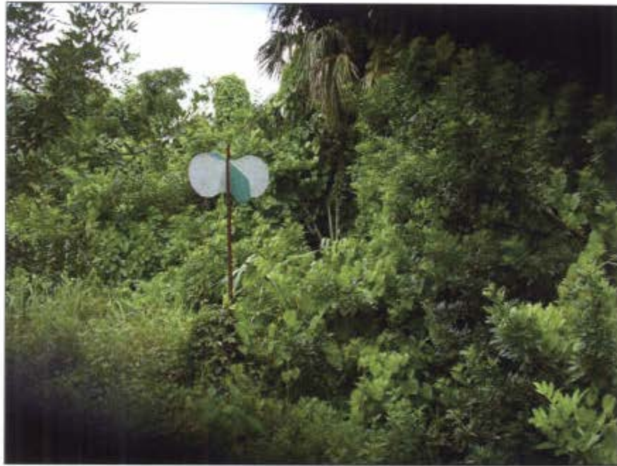
Figure 37. Photograph of railroad switch #3, facing southwest.
