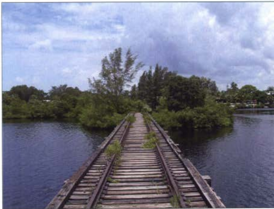
Figure 60. View of the deck of the timber trestle Railroad Bridge over Roberts Bay (8SO5293), facing north.
