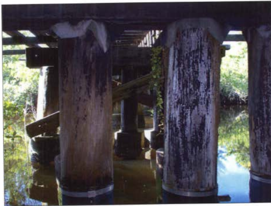
Figure 71. View of replacement piles of 8SO5314, placed on concrete bases, facing south.
