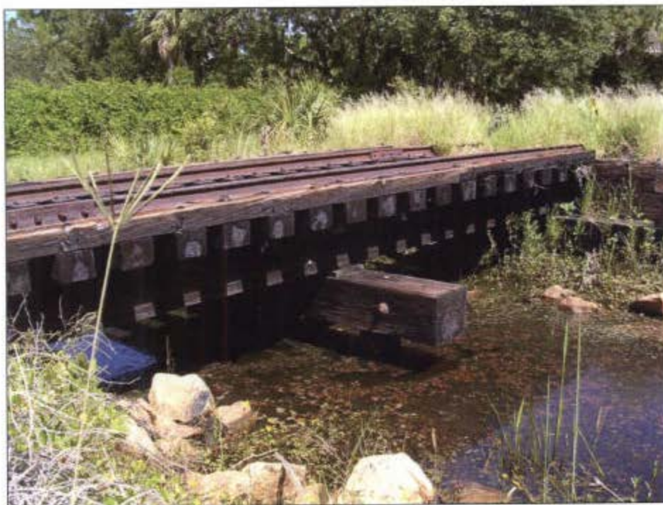
Figure 73. The substructure of 8SO5315, showing a long cap resting on 2-4 very short piles, supporting the deck, facing northwest.
