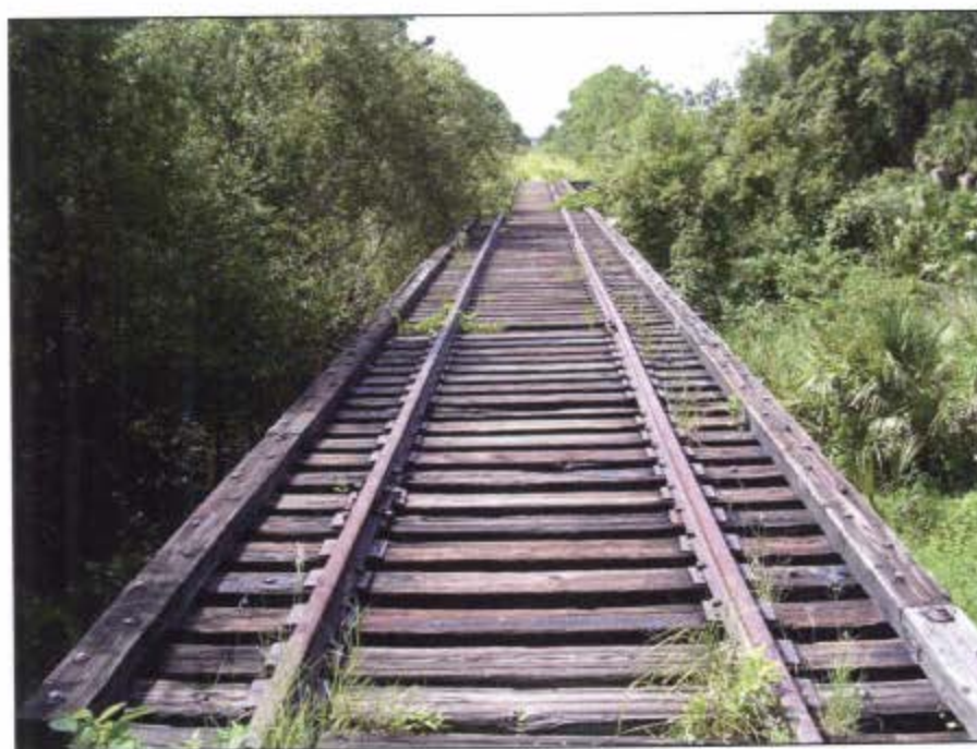
Figure 68. The long deck of 8SO5313, with the overpass for Highway 681 in the distance, facing south.
