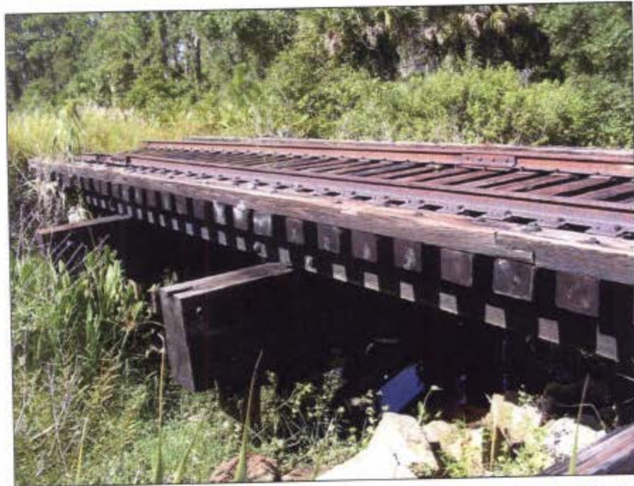
Figure 66. Double, stacked cap of 8SO5312, supporting the stringers and deck of the bridge, facing southwest.
