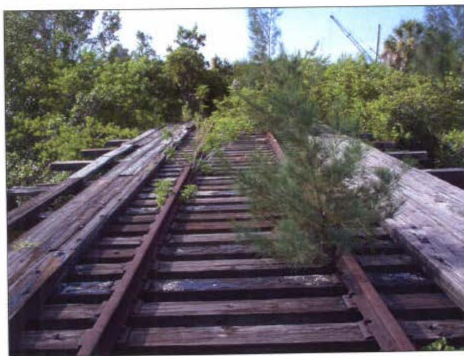
Figure 70. Deck of 8SO5314, with plank walkways on either side of the rails, facing south.
