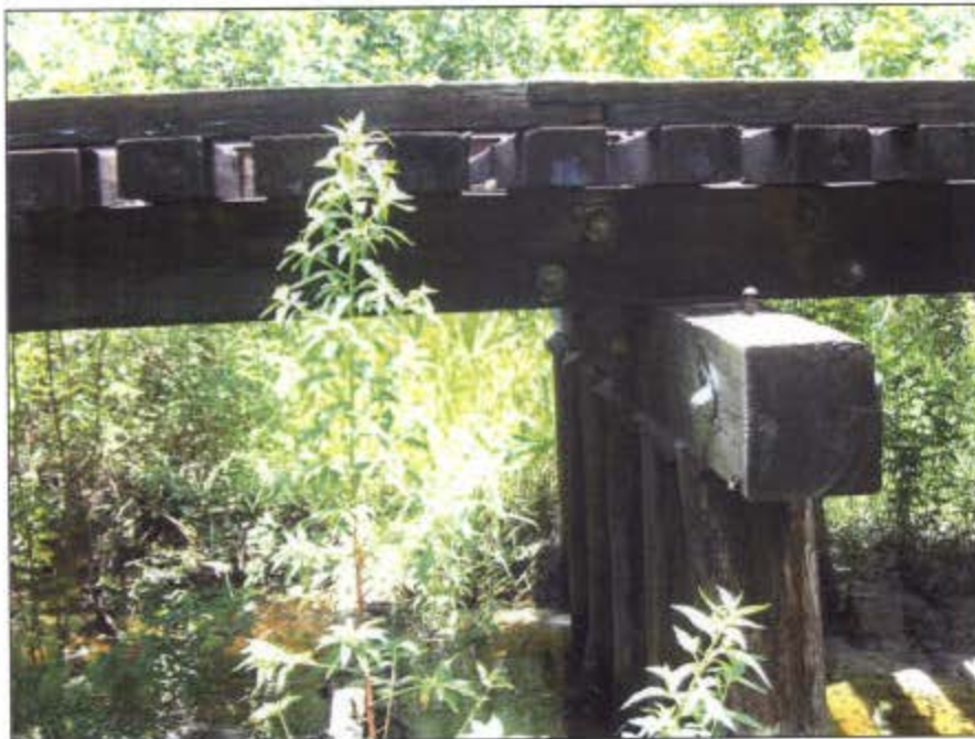
Figure 64. Bent with round piles of 8SO5310, facing west.
