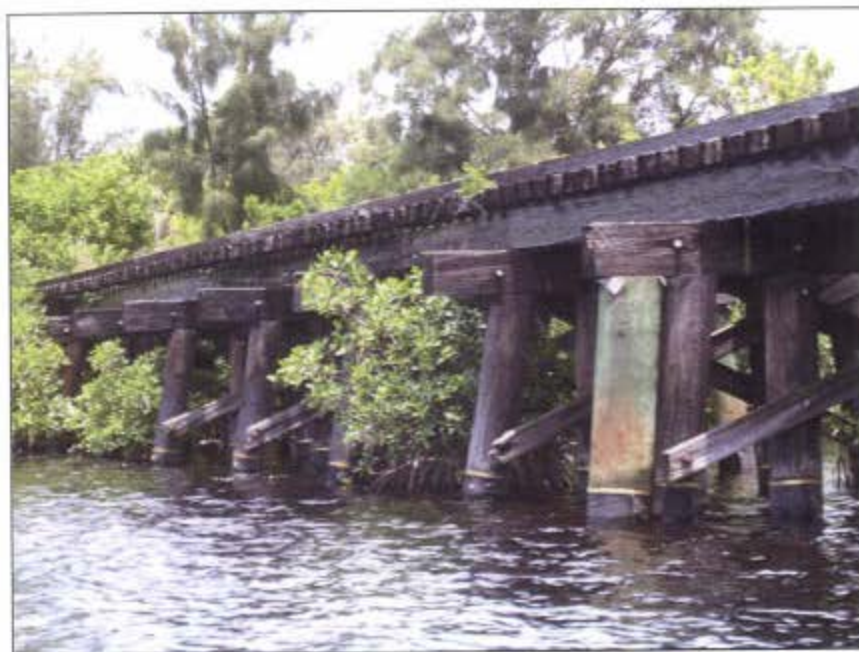
Figure 61. View of the north end of the Railroad Bridge over Roberts Bay (8SO5293), showing the round piles wrapped in rubber and the high tide mark, braced bents, bolted caps, stringers, and deck, facing northeast.
