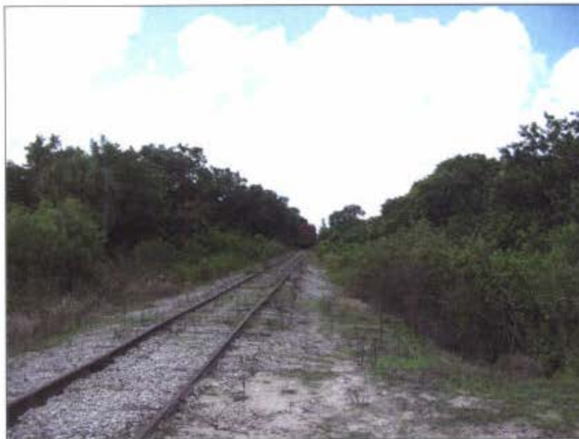
Figure 43. Photograph of railroad tracks in northern portion of project area, facing south.
