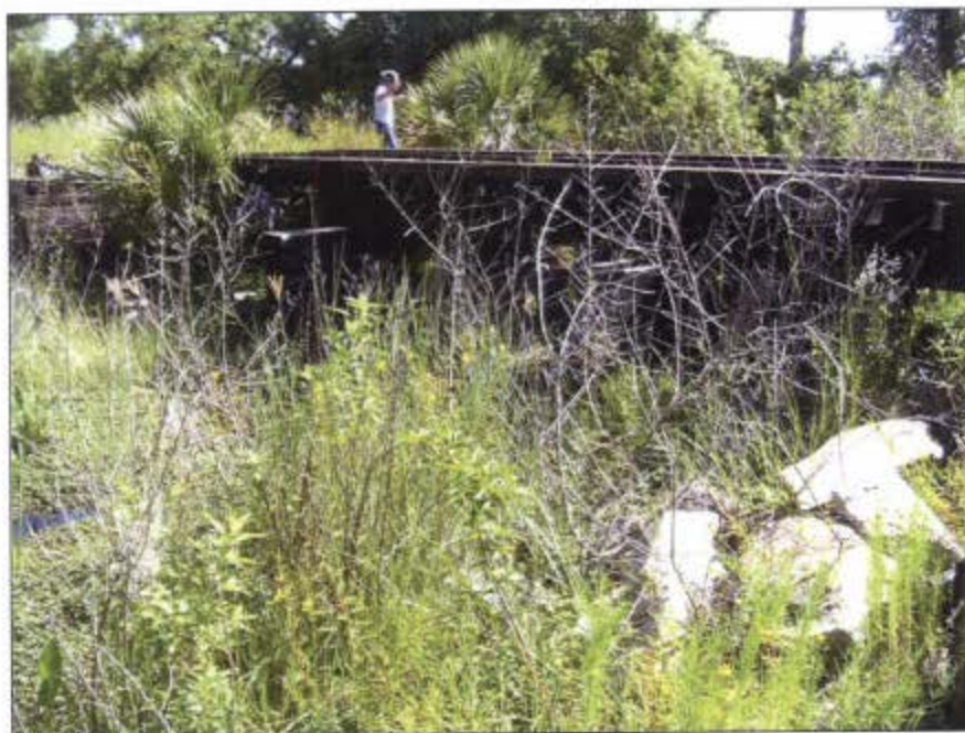
Figure 67. View of 8SO5312, showing bridge with a small stream running beneath it in an area overtaken by vegetation, facing northeast.
