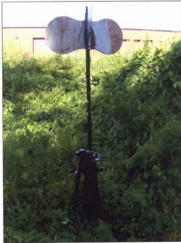
Figure 33. Photograph of railroad switch #1, facing west.
