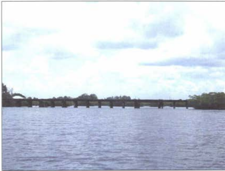
Figure 59. View of the open deck, timber trestle Railroad Bridge over Roberts Bay (Curry Creek) (8SO5293), facing west.
