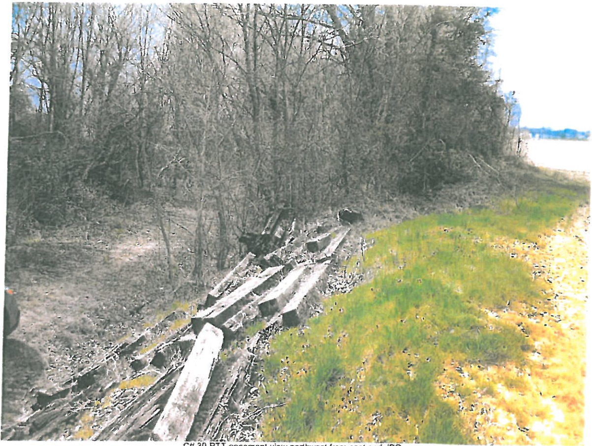
C# 39 RTT easement view northwest from east end.JPG 04/16/2018
