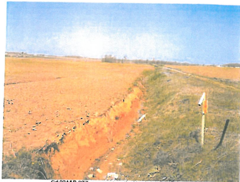
C# 22A&B RTT easement south side view northwest.JPG 04/18/2018
