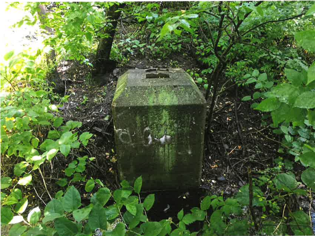
Photo 4. The south side block of the second set of catenary foundation blocks.
