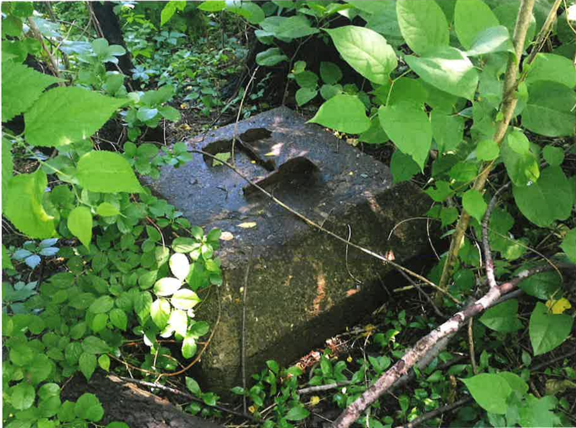
Photo 1. Foundation block for a catenary pole on the north side of the rail bed.
