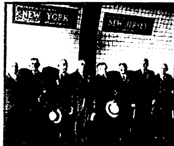
Build a tunnel and they will come. New York met New Jersey in the Holland Tunnel in 1927, and traffic quickly followed.
