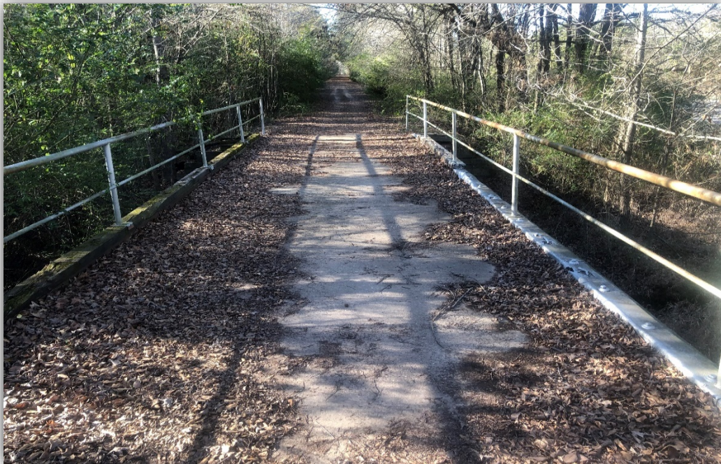
Section approaching a Wooden Trestle Bridge near Milepost 36.7 looking west
