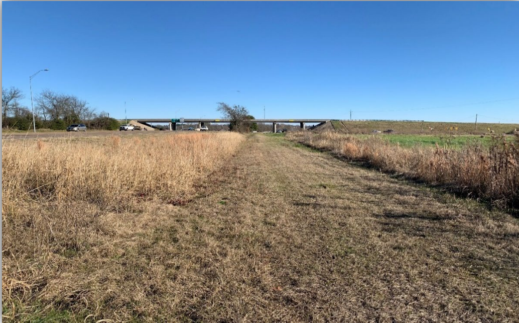
Section approaching De Kalb near Milepost 35.9 looking east at the US 259 Overpass
